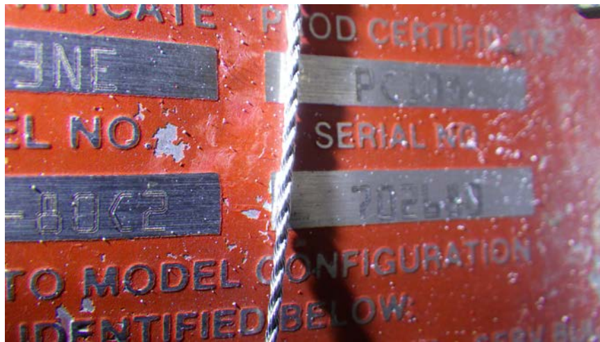
Photo No. 4: A data plate from one of the engines confirming the engine SN as 702680. (GE)
