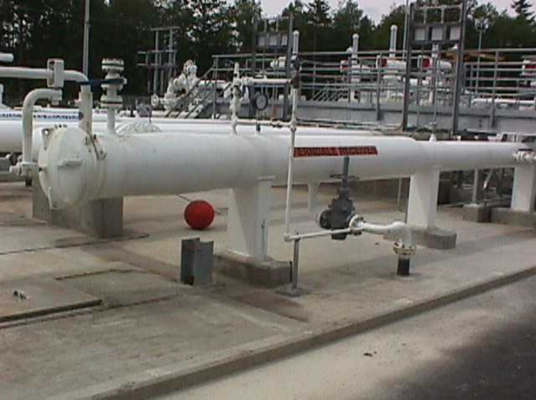
Appendix T to the Pipeline Operations Factual Report, Photo 3, Inlet receiver at Bayview.
