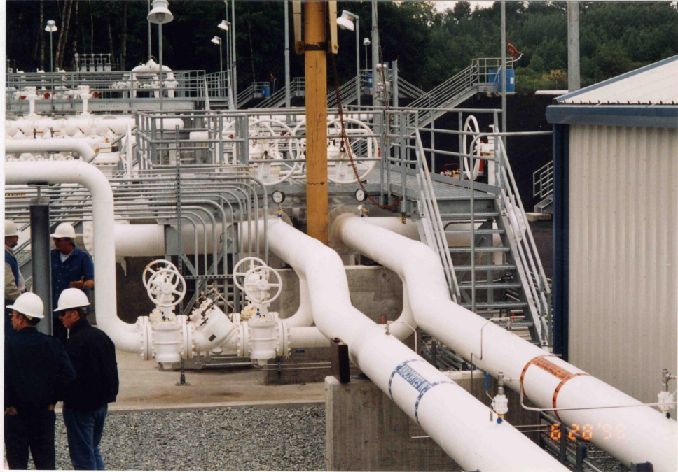
Appendix T to the Pipeline Operations Factual Report, Photo 2, RV-1919 connection to incoming pipeline.
