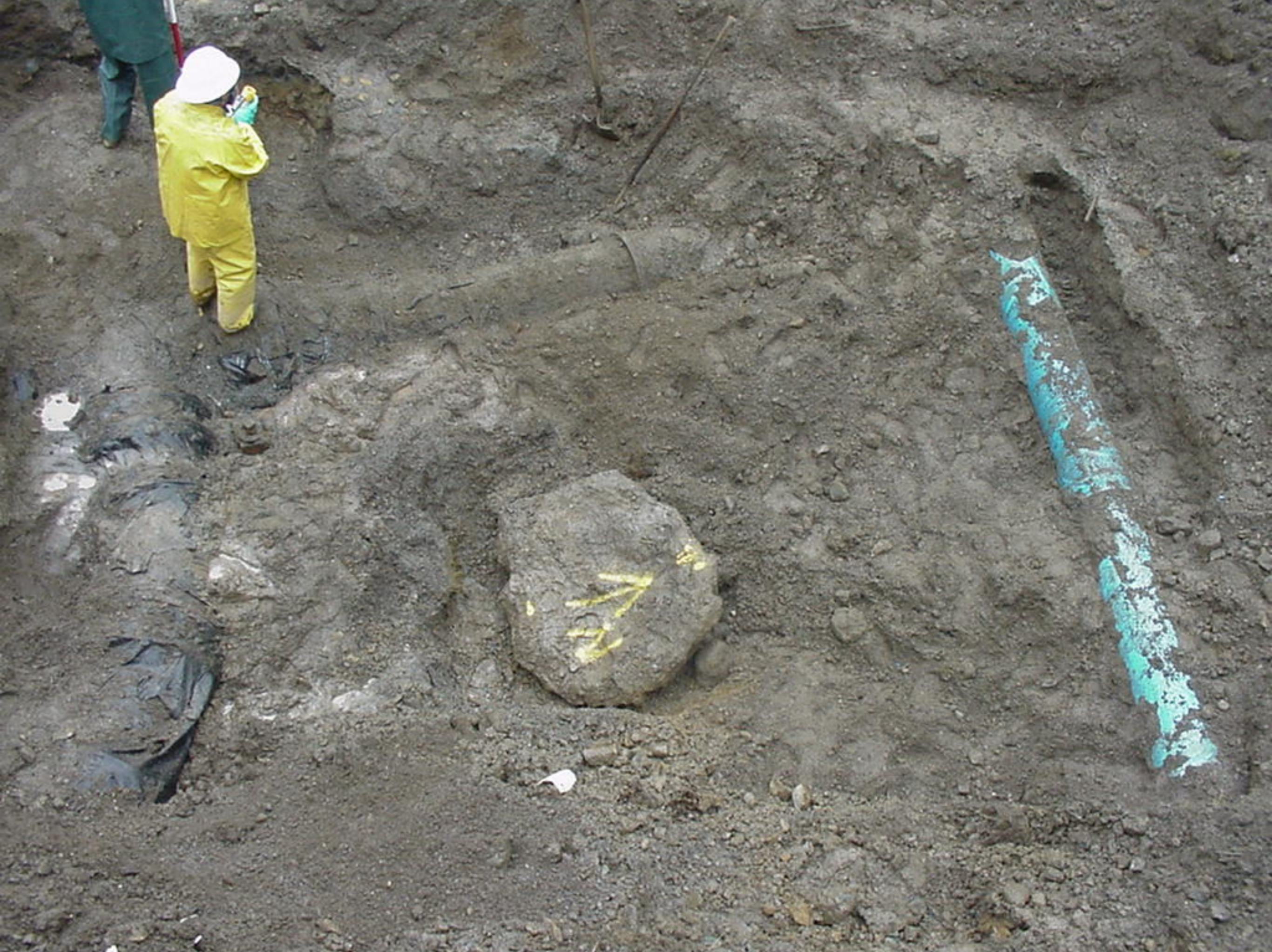
Appendix S to the Water Treatment Plant Factual Report, Photo 3, Irregular shaped concrete chunk found above rupture.
