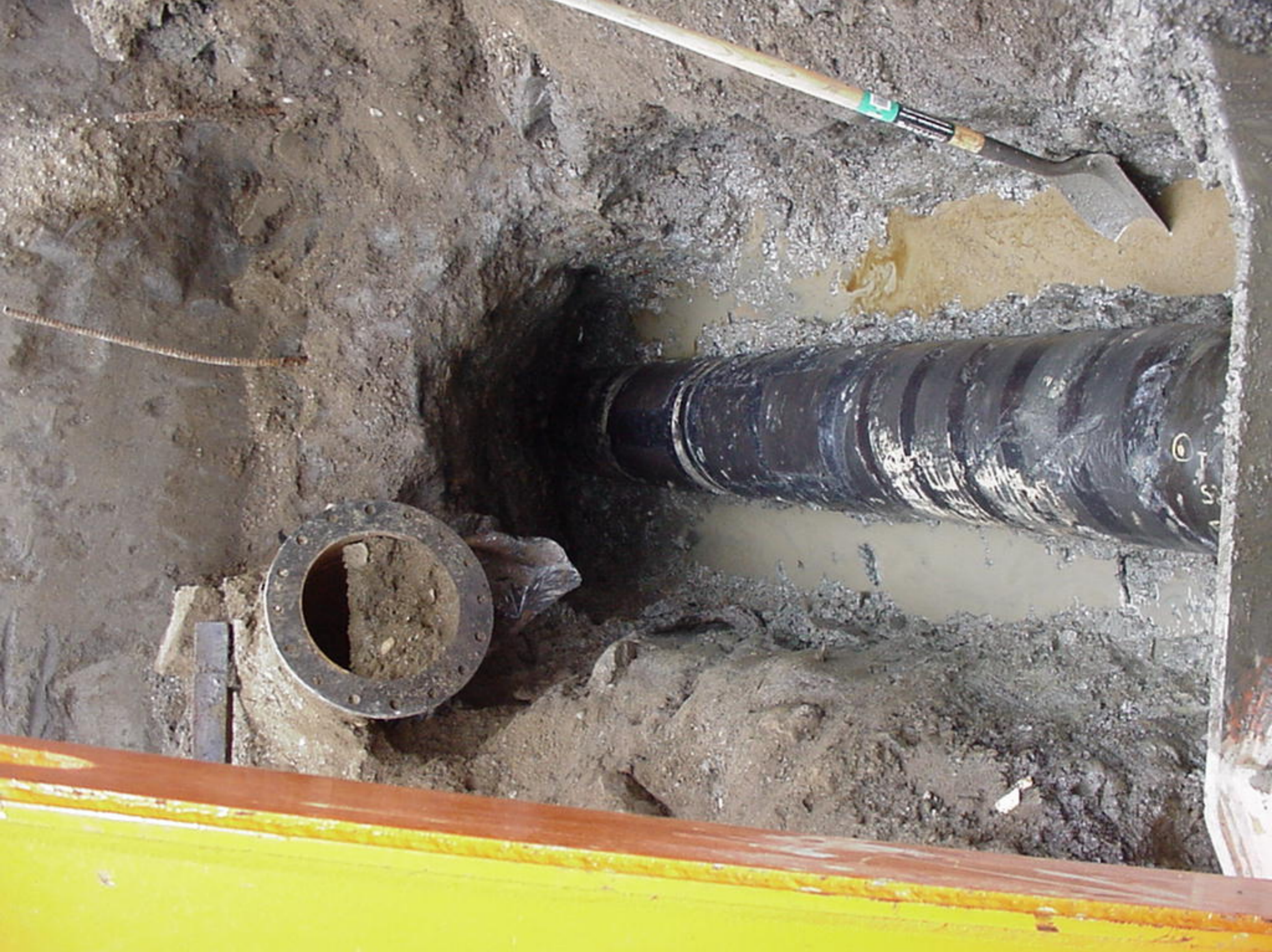
Appendix S to the Water Treatment Plant Factual Report, Photo 11, Second pipe segment with view of CDF fill that surrounds 72-inch waterline.
