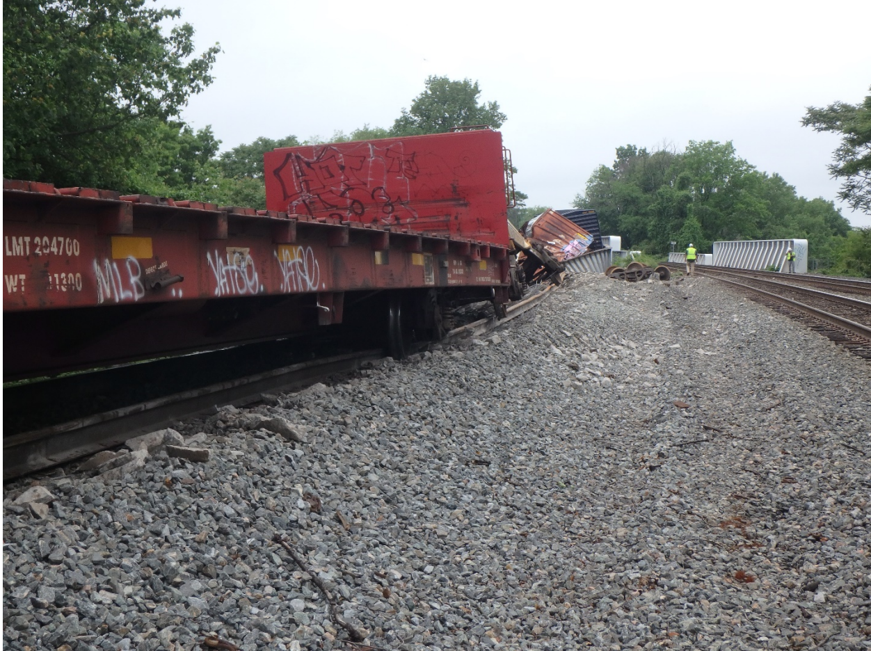
Figure 4. Photo showing track components damaged by wheel impact.
