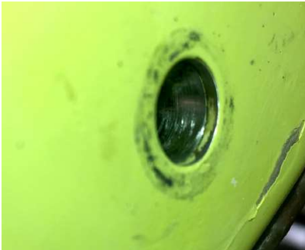
Figure A-6. The lower-right bolt hole. (Image courtesy of Arrow Aviation)
