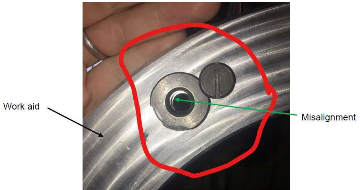
Figure A-4. Misalignment identified between the drill plate (work aid) and the upper-left longeron bolt hole. (Image courtesy of Bell)
