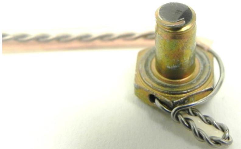
Figure 3 Fractured bolt isotropic view.
