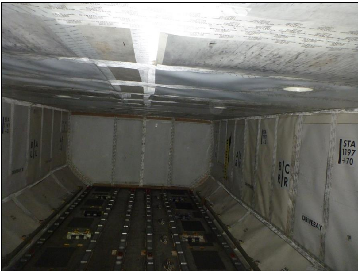
Figure 63 Aft cargo compartment (looking forward)
