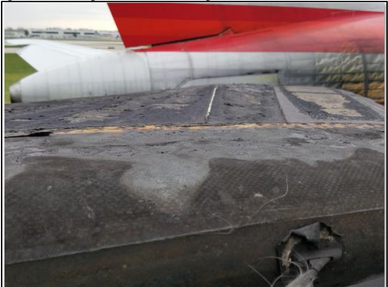
Figure 52 View of the right horizontal stabilizer looking inboard from the outboard end of the stabilizer
