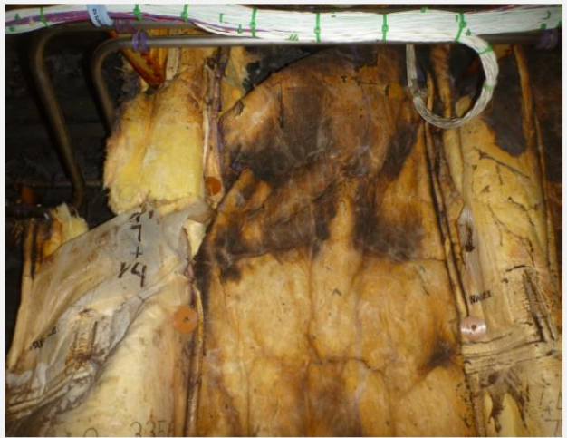
Insulation STA 1197+44 to 1197+66
