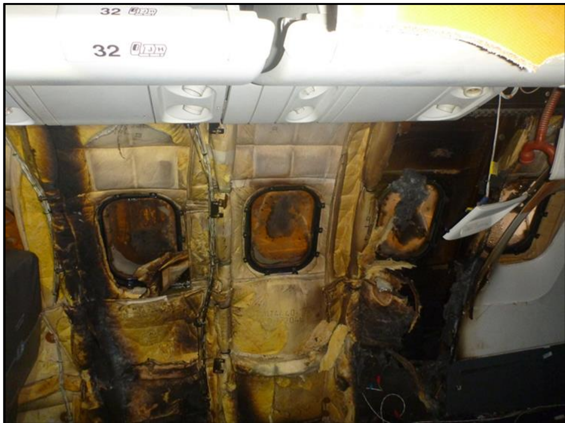
Figure 60 Charred insulation at seats 33 through 34
