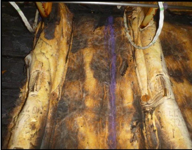
Insulation STA 1197+66 to 1197+88
