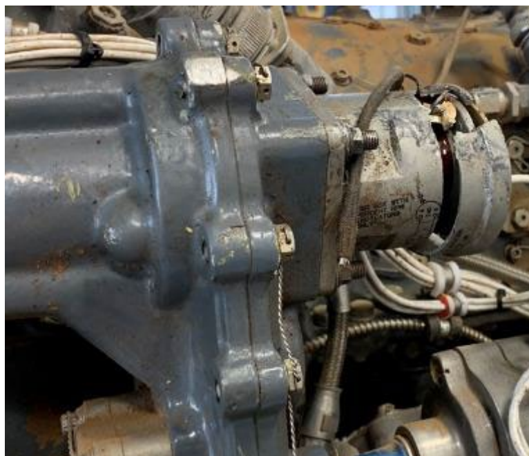
PHOTO 24: PARTIALLY FRACTURED N2-TACH GENERATOR HOUSING
