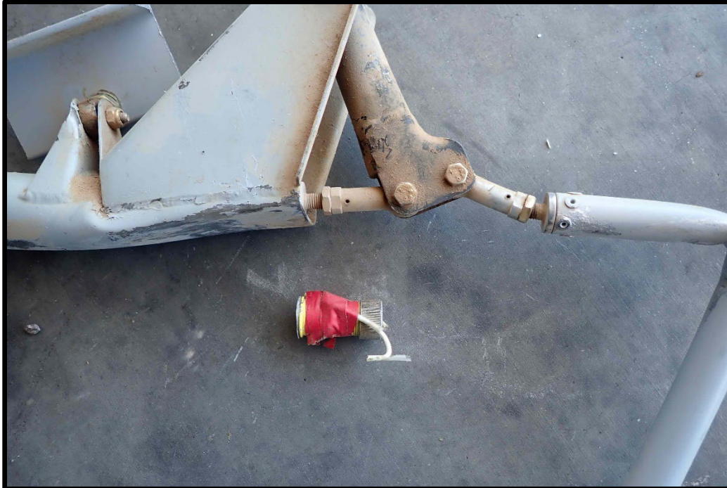
Figure 39 – Lamp socket and lower aft control column assembly
