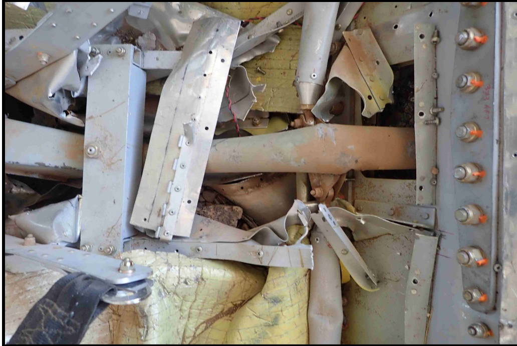
Figure 23 – Aileron push-pull tubes in underfloor
