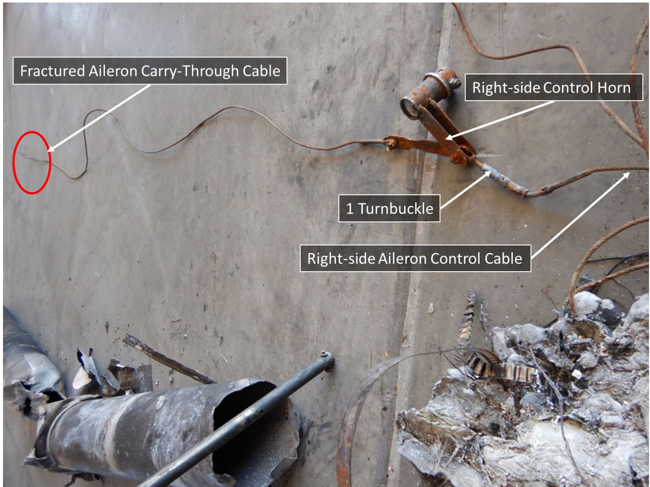
Figure 6. Image of the right-side aileron control cable system. The fractured end of the carry-through cable is circled in red.
