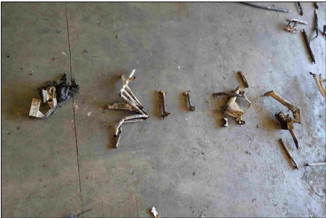
Photo 13 – Elevator Control System Remnants
