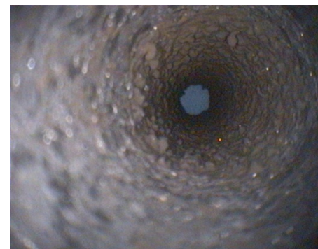
PHOTO 29: OIL VENT LINES
