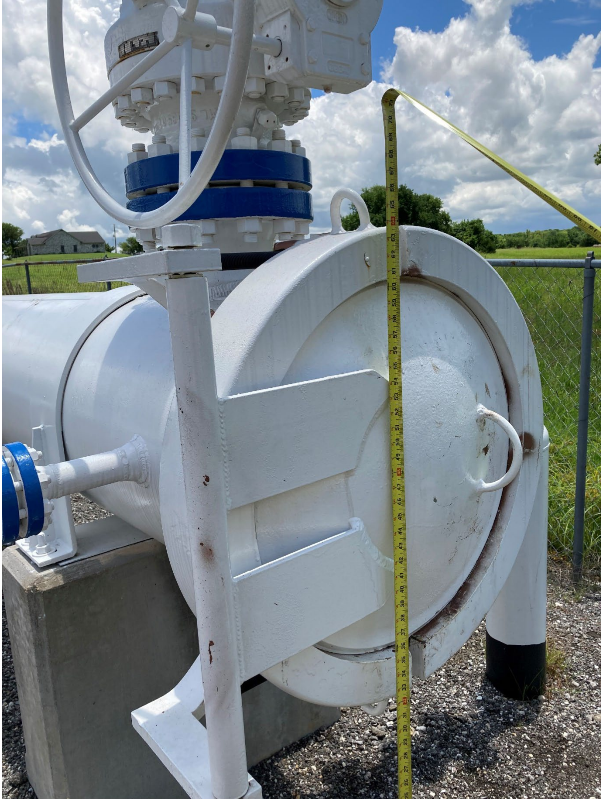
Figure 4. Launcher door (6/29/2021 at 1:17PM, Courtesy of RRC)
