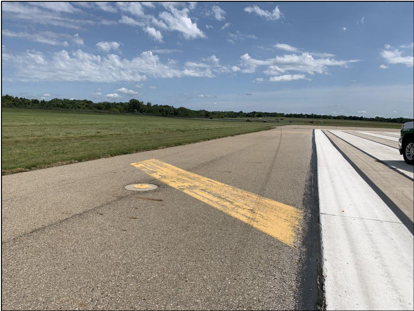
Photo 9 – Runway Skid Mark / Right Tire (FAA Photo)
