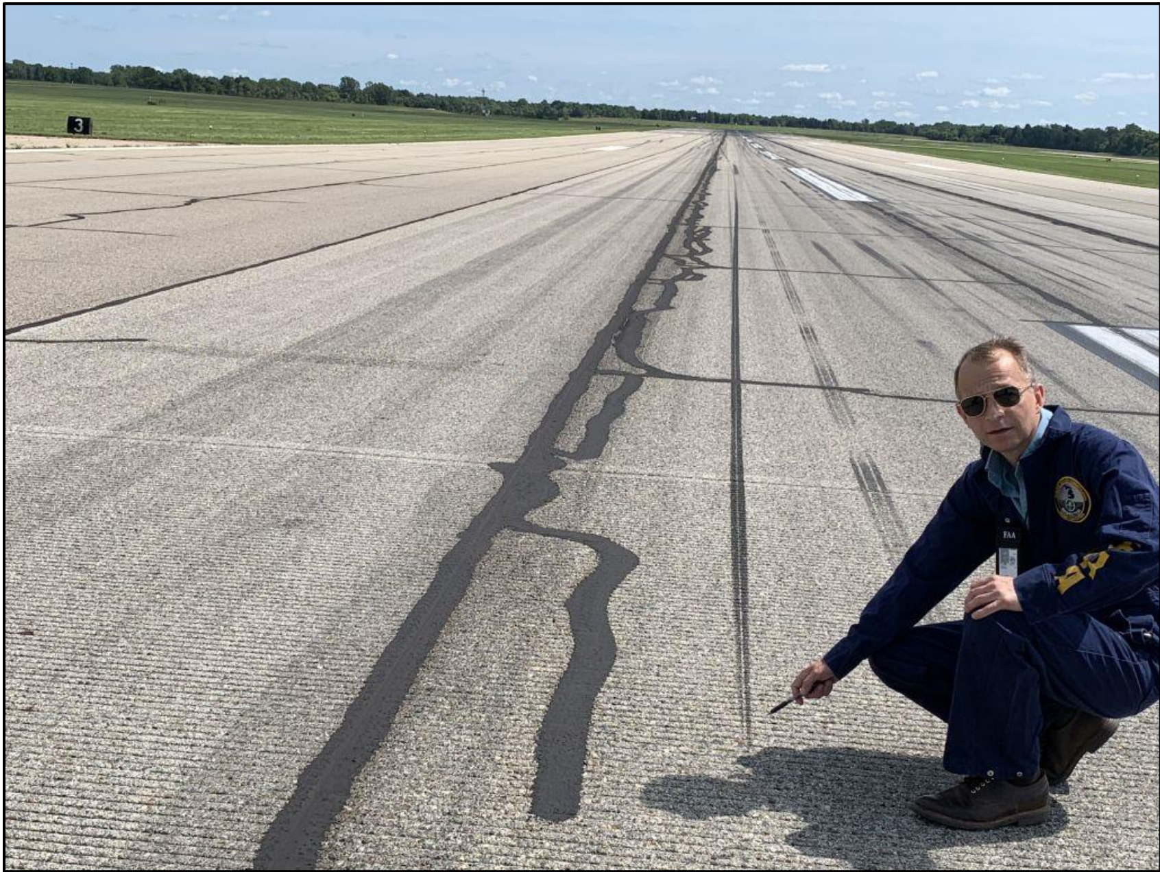
Photo 7 – Runway Skid Mark / Left Tire (FAA Photo)
