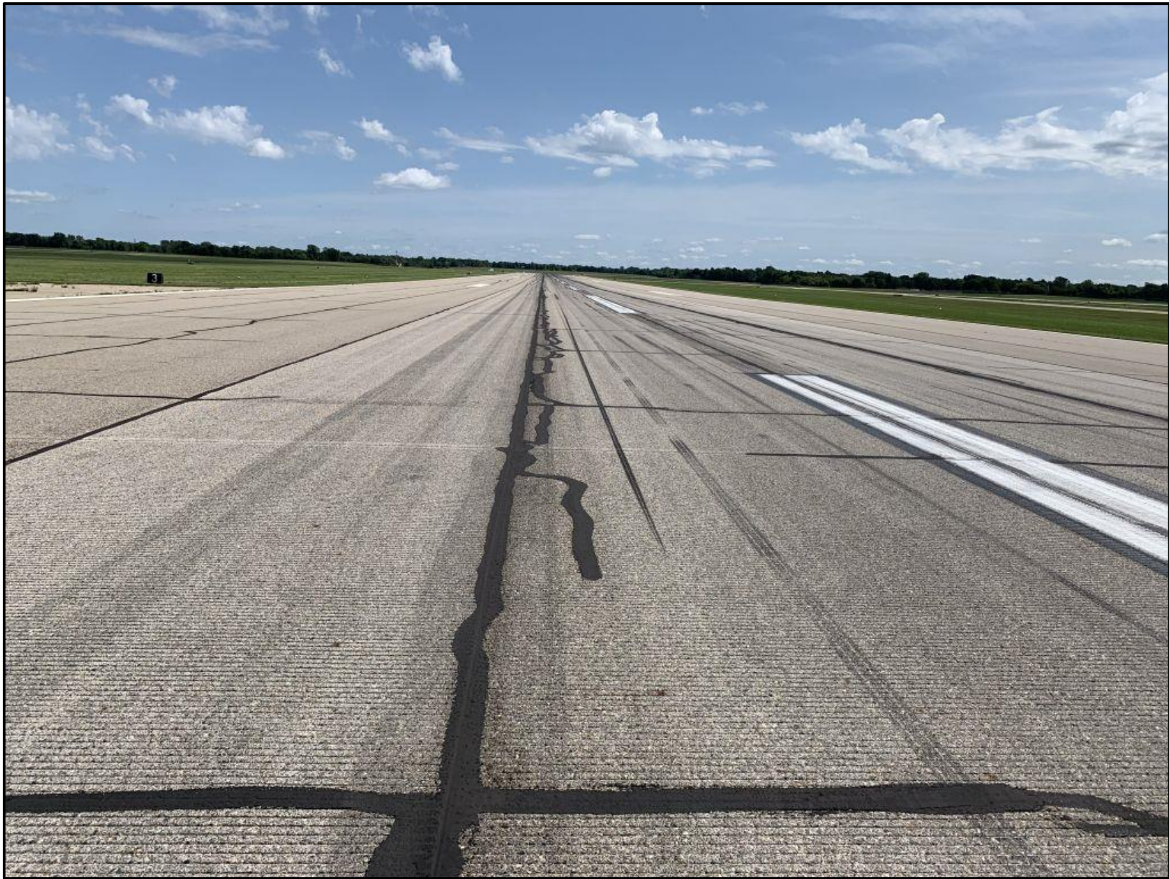
Photo 8 – Runway Skid Mark / Left Tire (FAA Photo)
