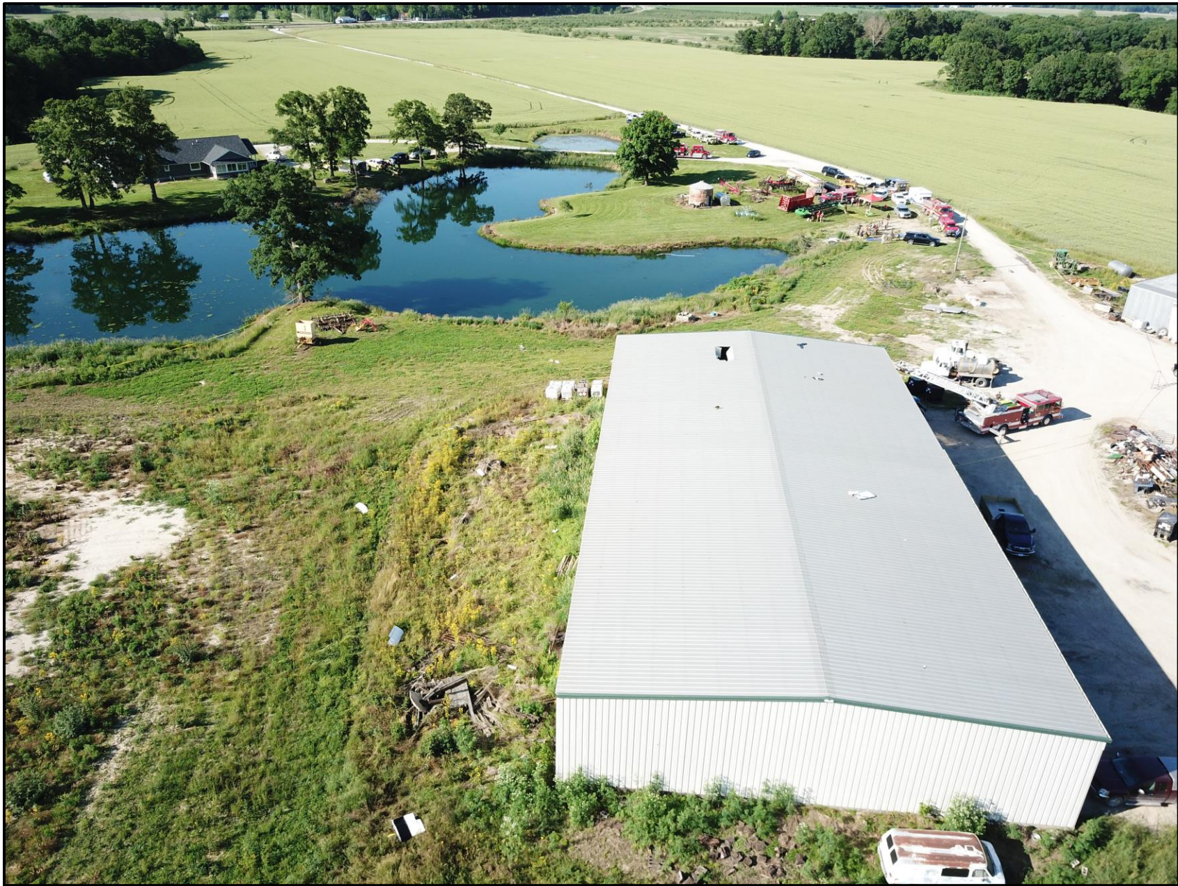
Photo 1 – Aerial View of Accident Site (Fire Dept Photo)
