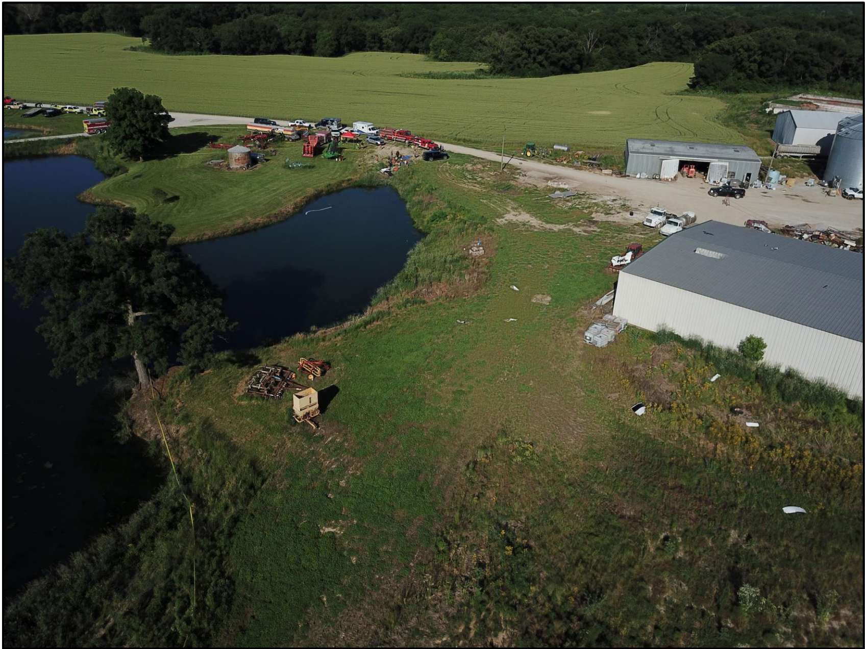
Photo 2 – Aerial View of Accident Site (Fire Dept Photo)
