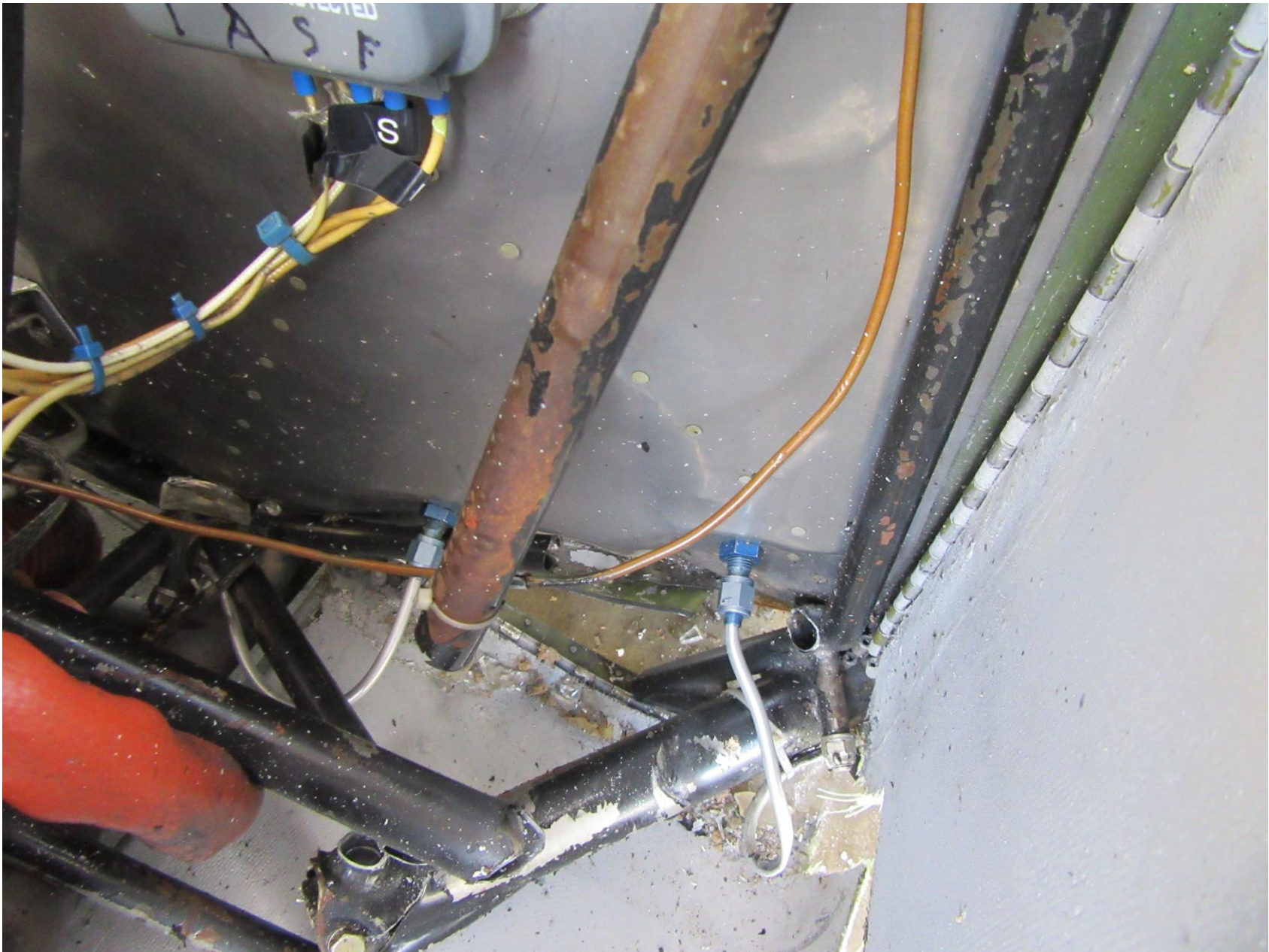
Photo 5 – Close up view of the substantial damage sustained to the engine mount (courtesy of the Federal Aviation Administration).
