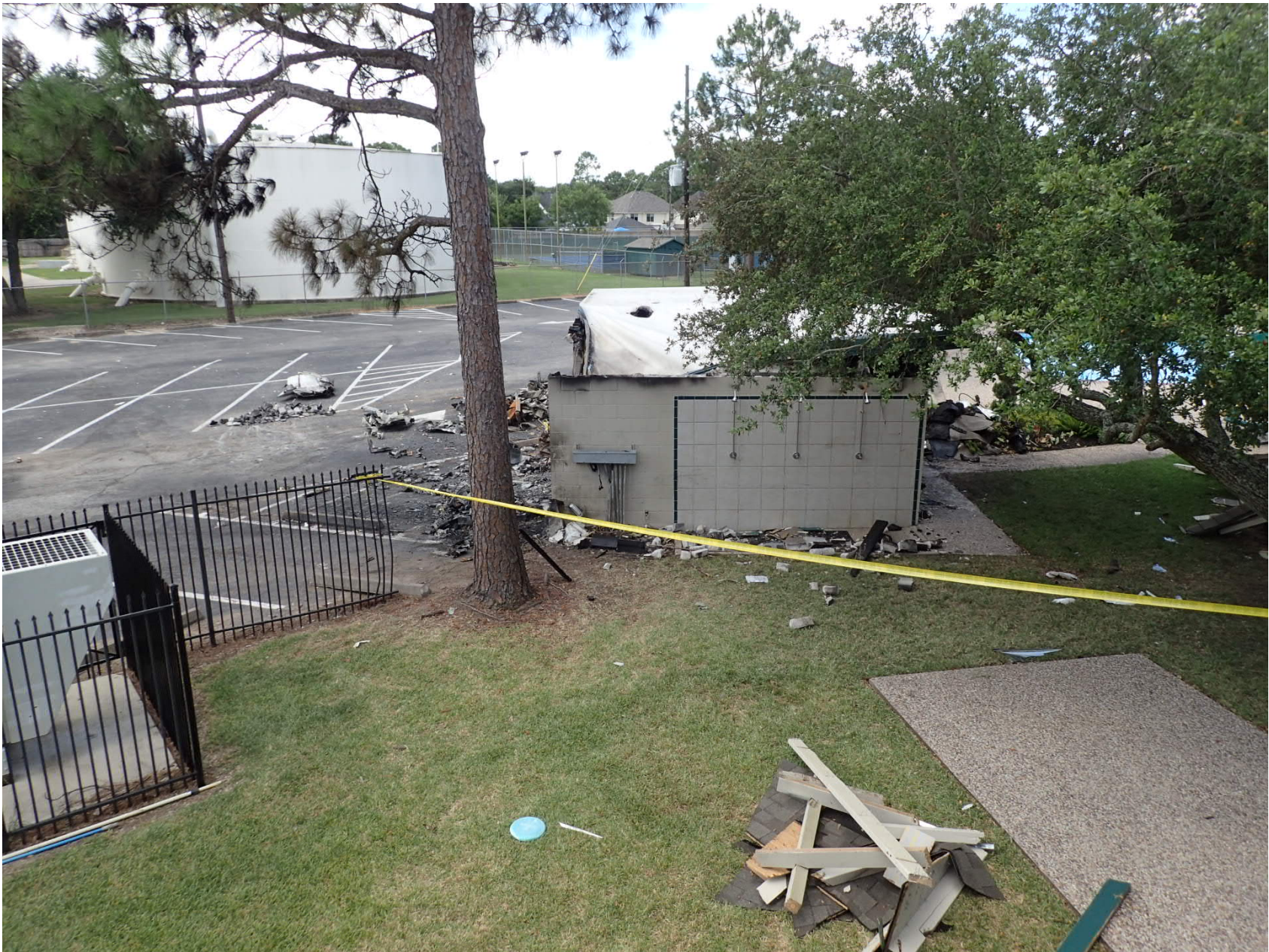
Photo 7 – View of the parking lot and the building.
