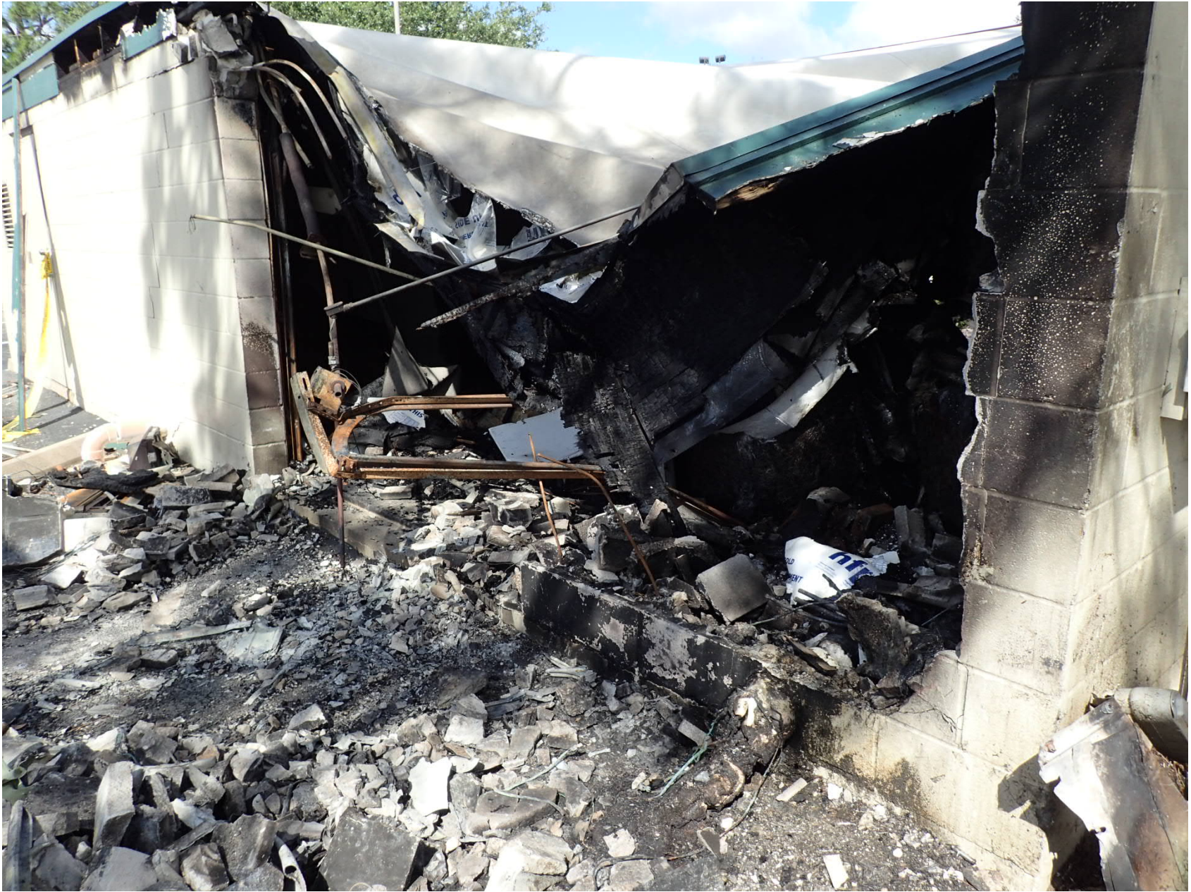
Photo 6 – View of the building.
