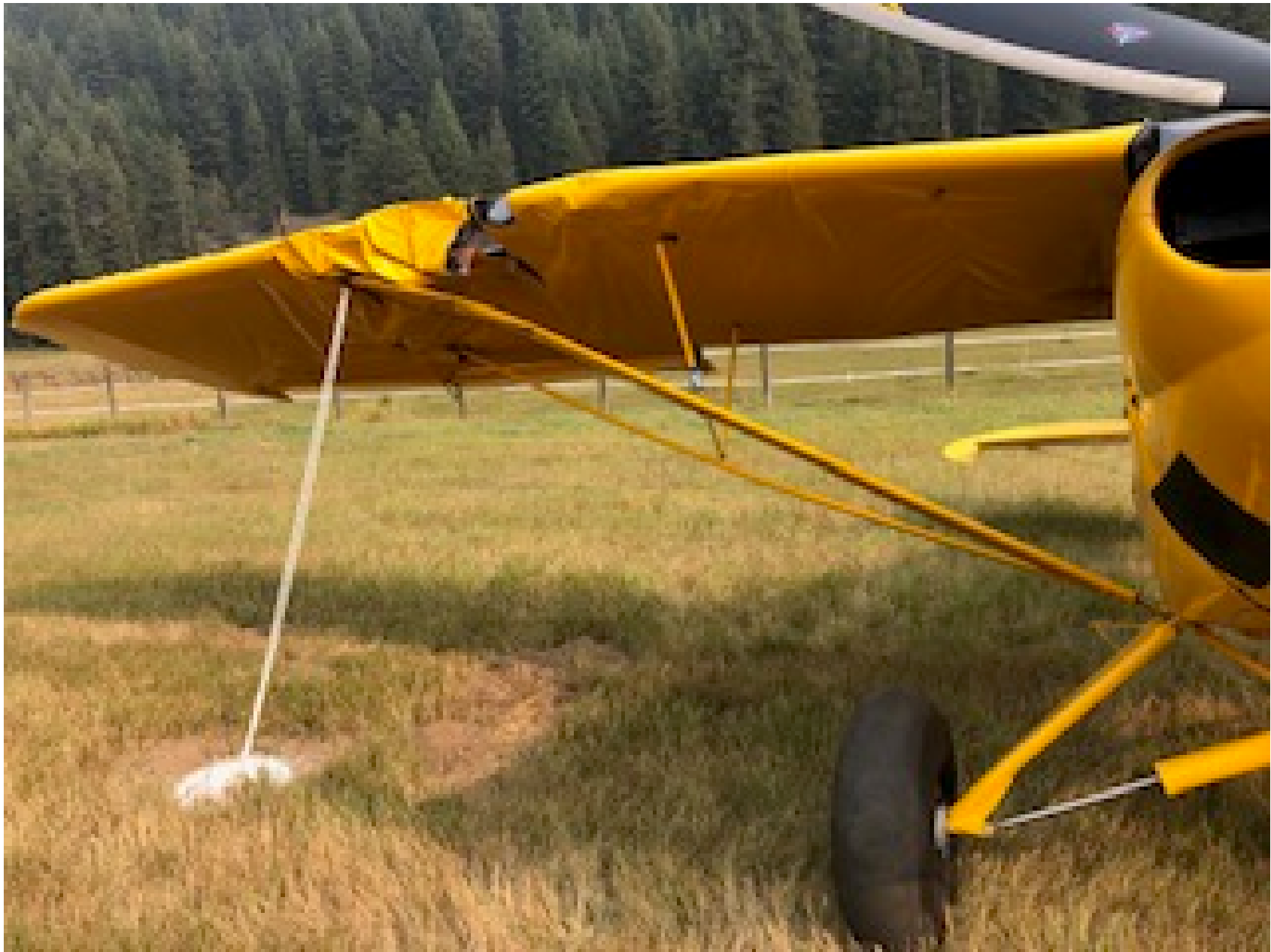
Photo 1 – View of damage to right wing and lift strut (courtesy of the pilot)
