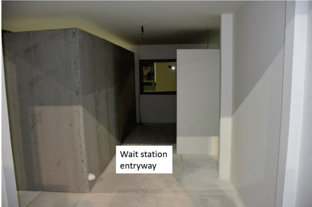
Figure 19: Phase 3, Test structure, hallway with direct line of sight to room of origin (361029_1336740. JPG)
