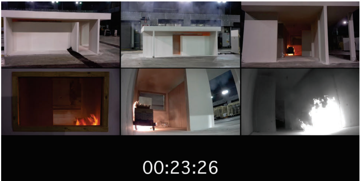
Figure 45: Phase 3, Test 1 (361029_Master_1345478)
