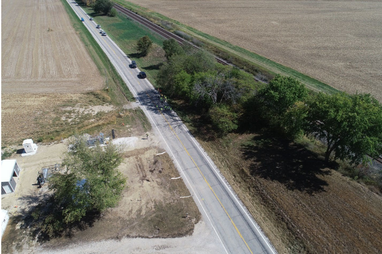
Figure 1. Aerial image of US Route 40 looking southeast.
