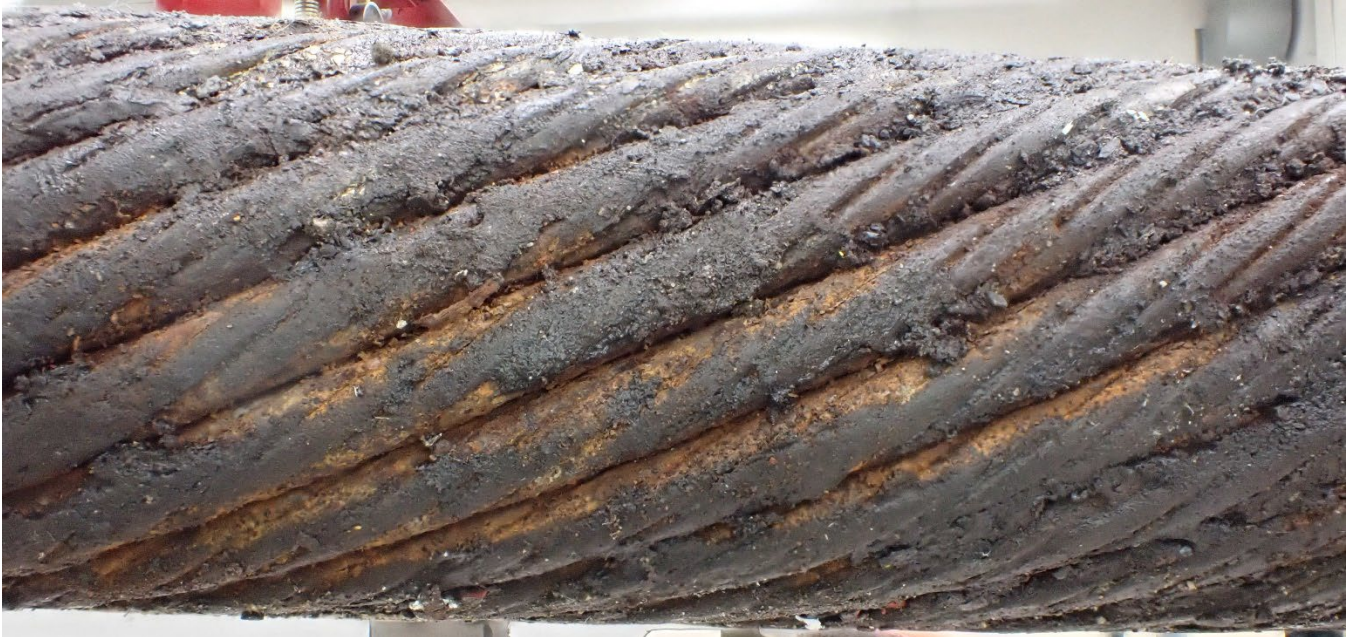
Figure 8 Representative image showing the rough surface and heavy corrosion product buildup observed on Specimen 2 (76, crane-side of fracture). (37-inches from reference end, Severity Rating 60%)
