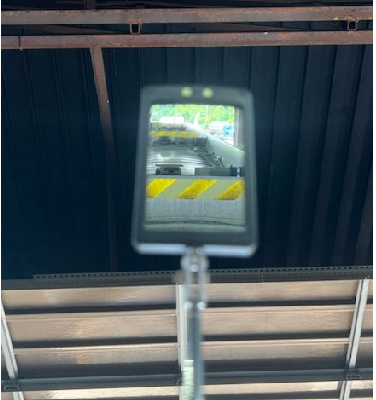
Figure 4 - View through inspection mirror (TK Transport)
