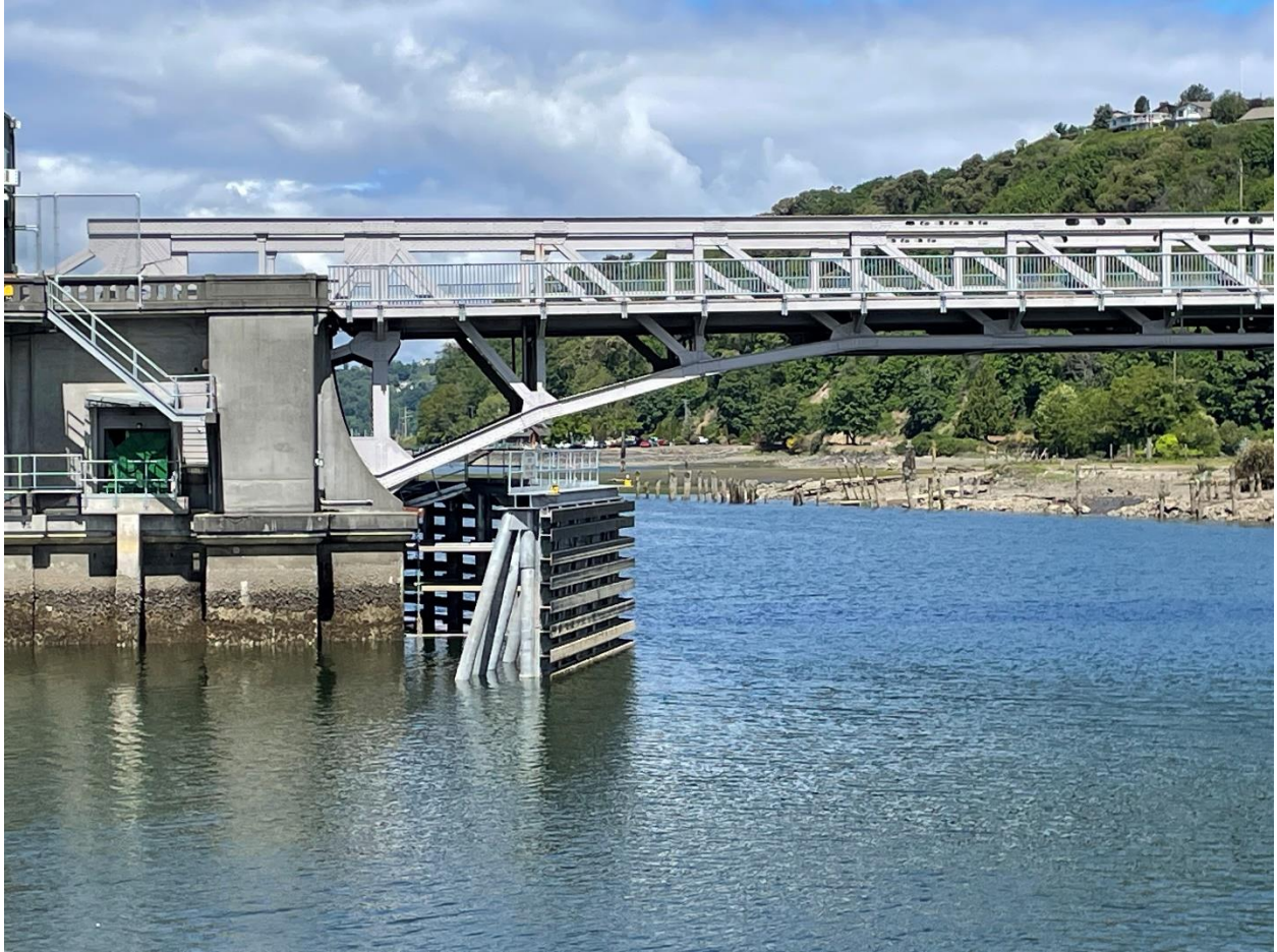
Close-up view of repaired Hylebos Bridge fender constructed of steel.
