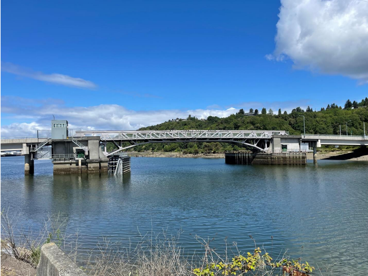
Hylebos Bridge post-repair.
