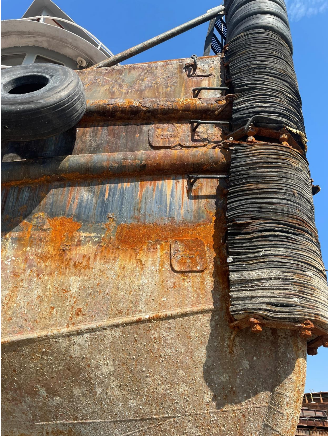
Doubler plates, starboard bow
