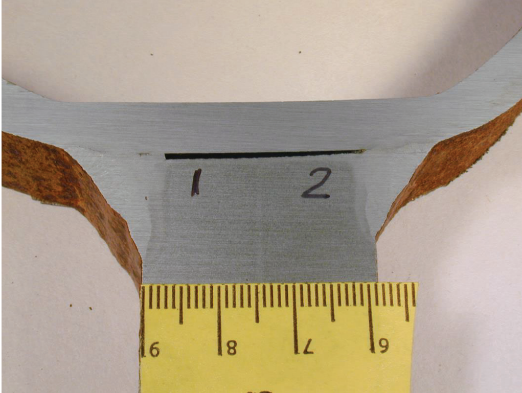
Fig. 27: Close up view of the etched weld x-section. Note, no defects were observed.
