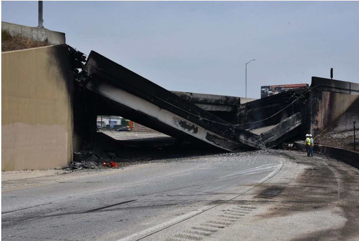
Figure 1. Post-crash view of scene. International truck underneath collapsed I-95 overpass. (Source: PSP)
