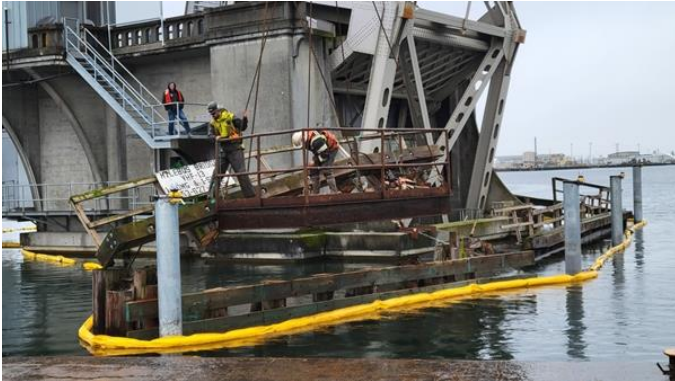
116. Inspecting catwalk prior to cropping
