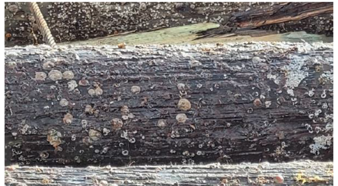
243. No 26 fender pile – visually generally satisfactory with light surface checking
