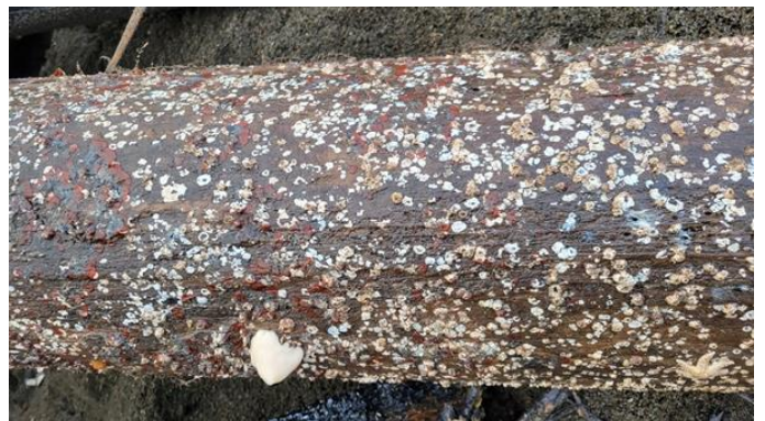
171. No 13 fender pile – satisfactory
