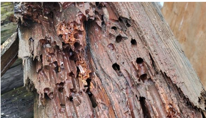
186. No 3 pile cluster – worm tracks
