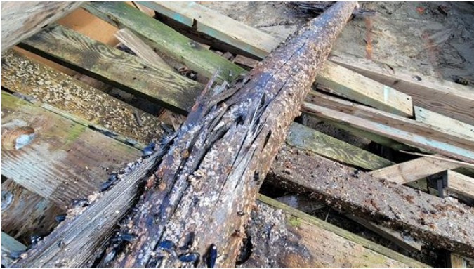
208. No 4 batter pile – checking over surface area
