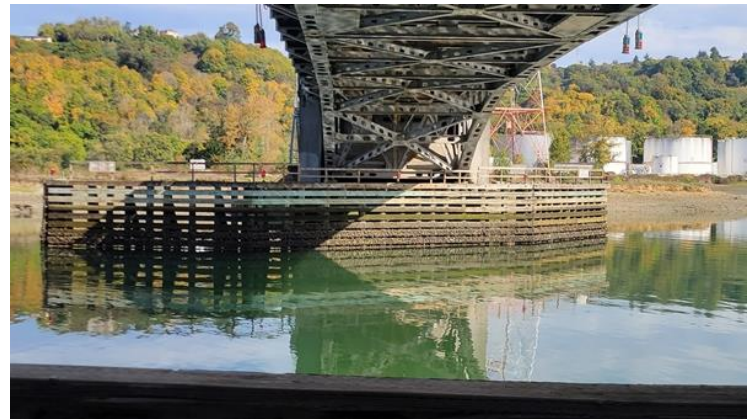
18. Undamaged east fendering
