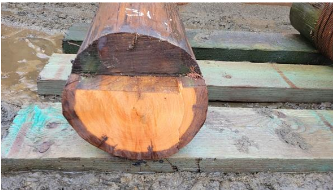
124. Top of pile No 31 – visually satisfactory
