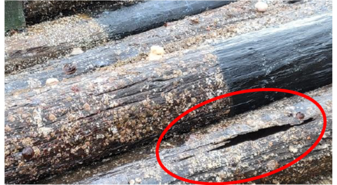
233. No 3 pile 4 th cluster – hollow core
