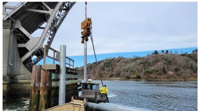
105. Driving 2 nd pile
