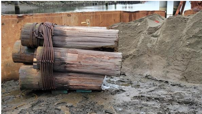
130. Top of No 4 cluster – general view
