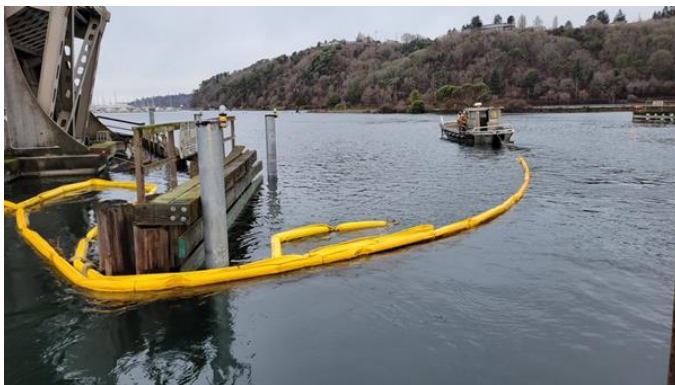
114. Deploy anti-pollution boom
