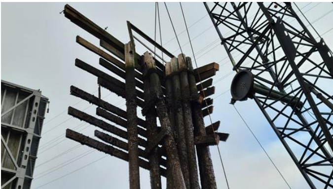
190. Lift and remove no. 2 pile cluster
