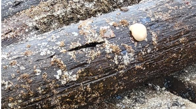
228. No 5 pile 4 th cluster – checking on surface.
