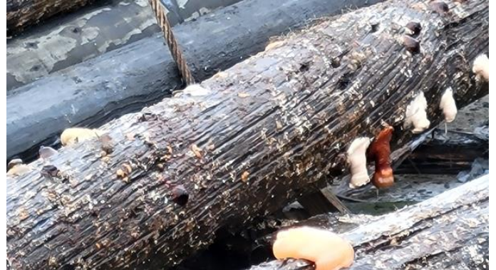
229. Center pile 4 th cluster – heavy worm tracks
