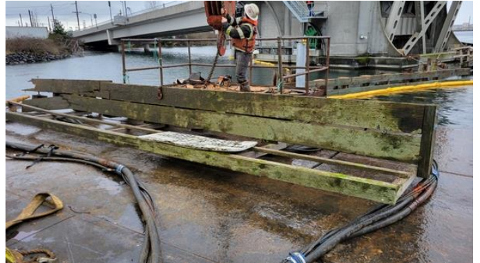
117. Inspecting catwalk prior to cropping
