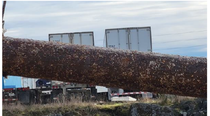
245. No 24 fender pile – visually generally satisfactory
