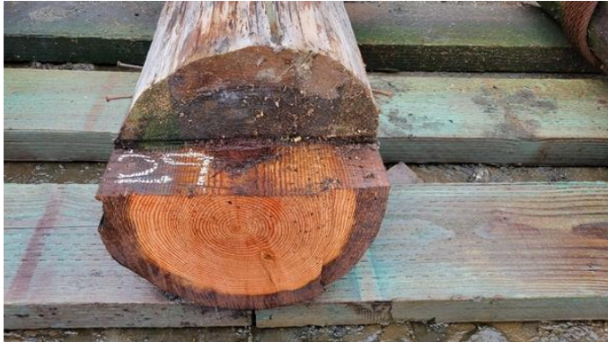
126. Top of Pile No 29 – visually satisfactory
