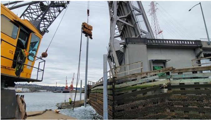
110. 6 th Pile in position
