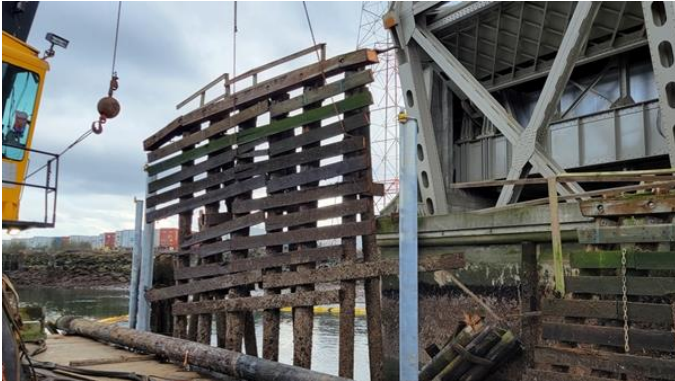
134. Rear section – center wing wall – being lifted
