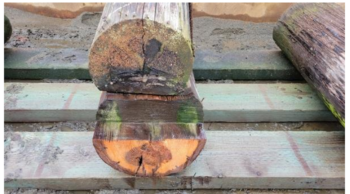
125. Top of pile No 30 – rotting of core section
