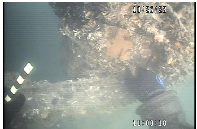
30. No 1 C batten remains
