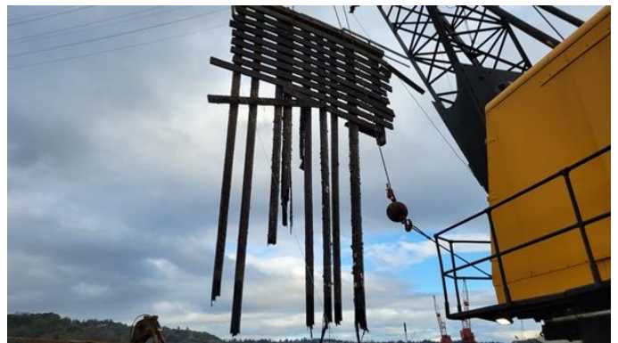
161. Center wing wall removal
