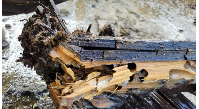
213. No 1 cluster pile – core degradation and extensive worm tracks o 24 fender pile – visually generally satisfactory
