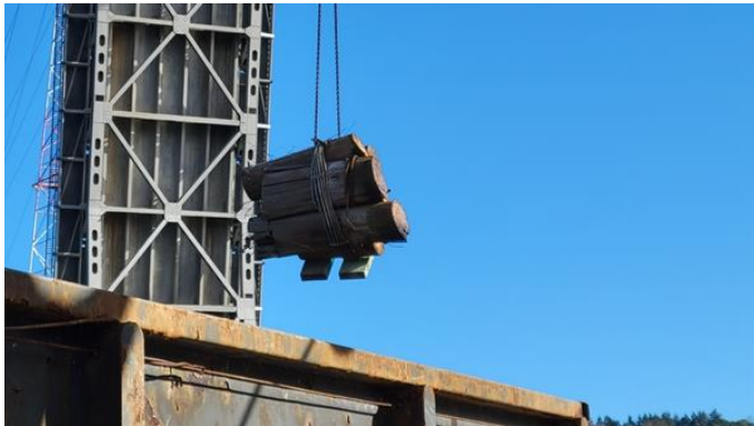
200. North wing wall top section removal
