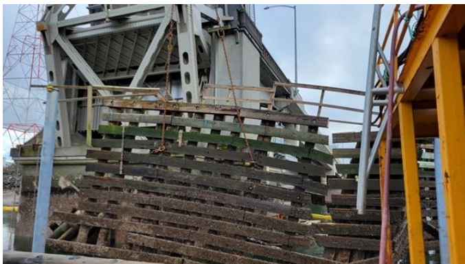
160. Center wing wall removal
