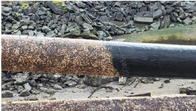
244. No 24 fender pile – visually generally satisfactory
