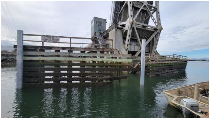
106. 1 st And 2 nd piles in position
