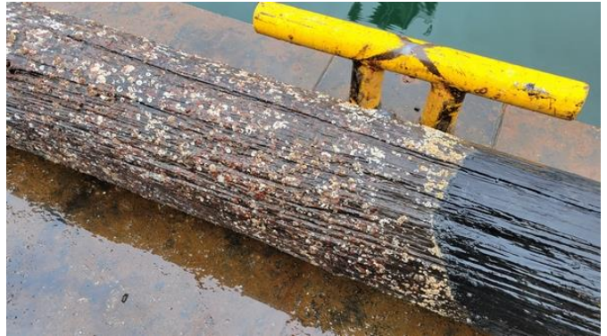
123. Pile 25 – surface checking
