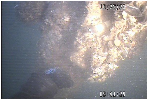
61. No 4 pile – horional with core loss
