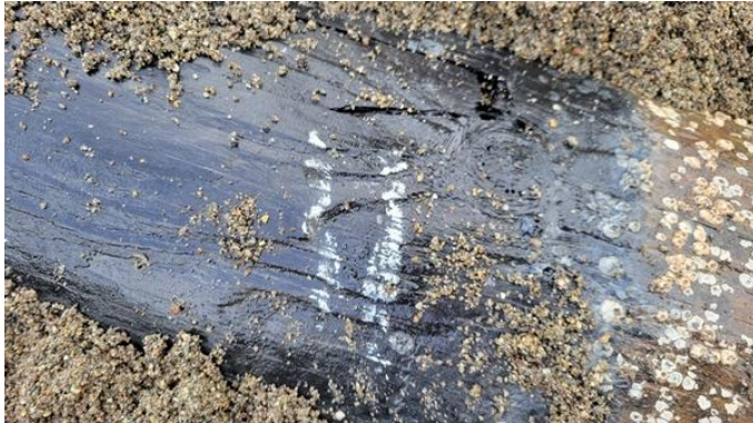
166. No 11 fender pile – satisfactory
