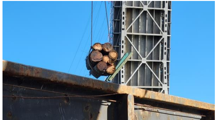
201. North wing wall top section removal
