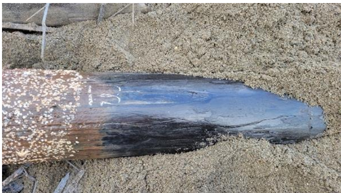
170. No 13 fender pile – satisfactory
