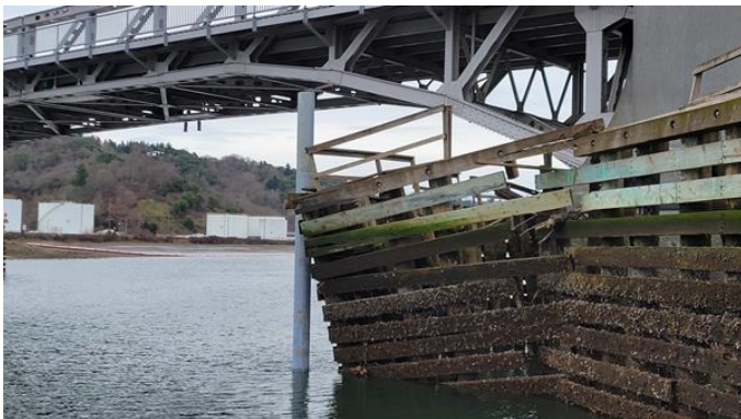
108. 4 th Pile in position
