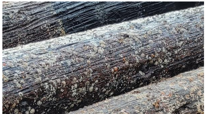
239. No 29 fender pile – generally satisfactory with light surface checking
