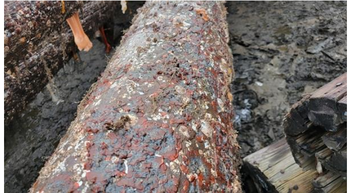
167. No 11 fender pile - satisfactory
