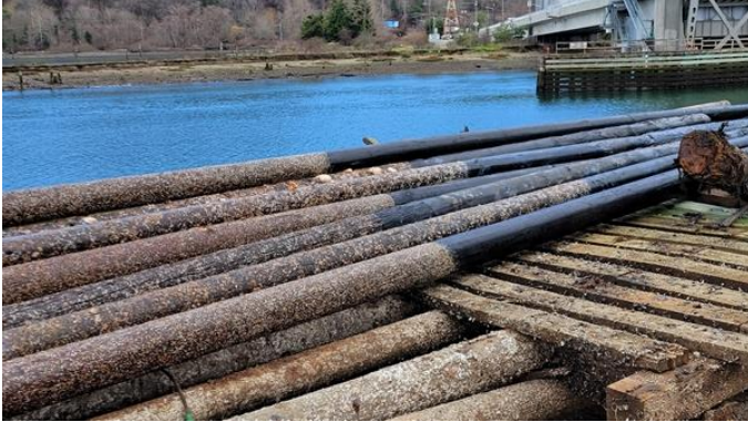
216. Pile Nos. 1-6 loaded on barge
