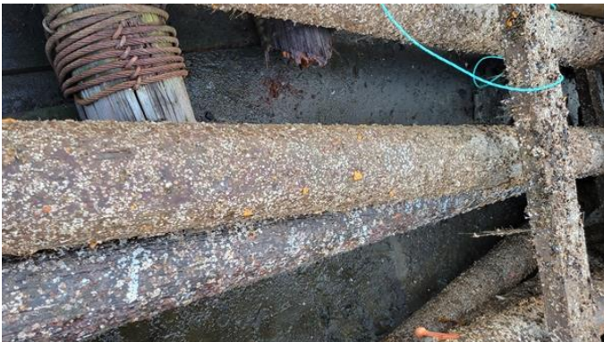
178. No 16 fender pile – satisfactory
