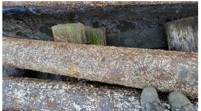
179. No 16 fender pile – satisfactory
