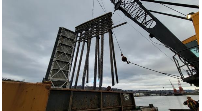
135. Rear section – center wing wall – being lifted
