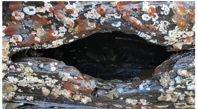
215. No 1 cluster pile – hollow core
