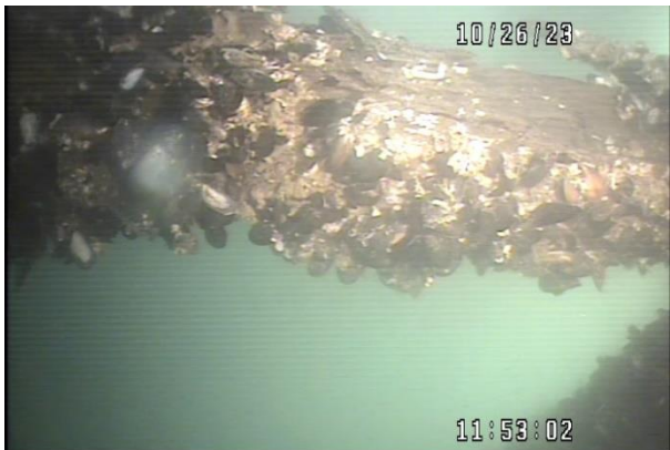
41. No 6 pile – south support
