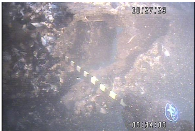
57. Batten 2A – 90% section loss on end
