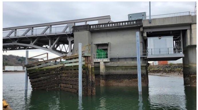
109. 5 th Pile in position
