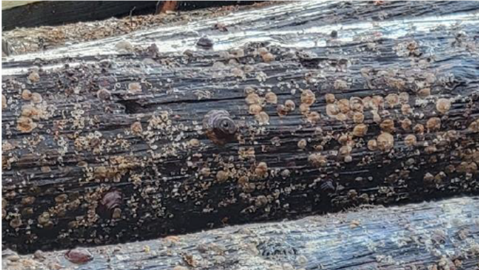
240. No 28 fender pile – generally satisfactory with light surface checking
