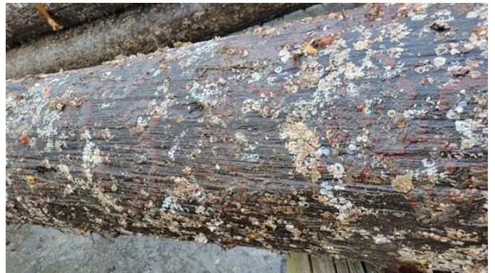
155. Pile No 22 – surface checking
