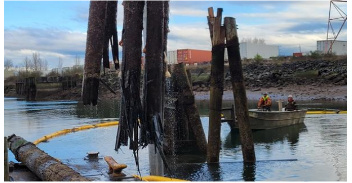
183. Remove No 3 pile cluster
