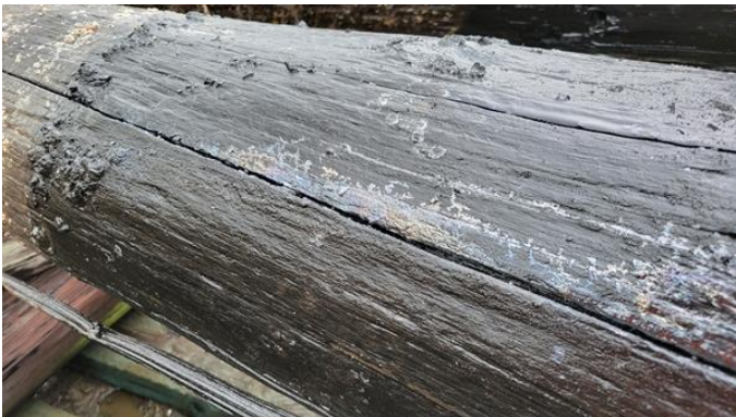
154. Pile No 22 – surface checking
