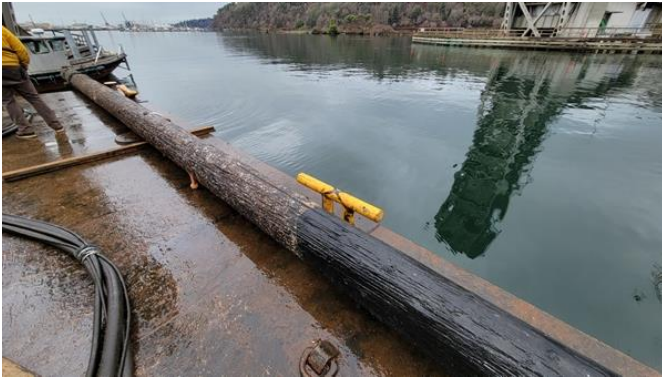
122. Pile No 25 on barge
