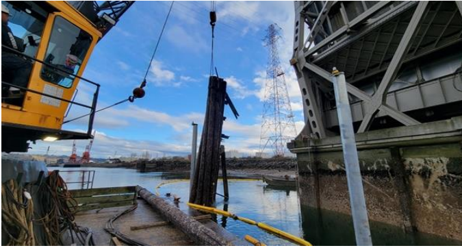
182. Remove No 3 pile cluster
