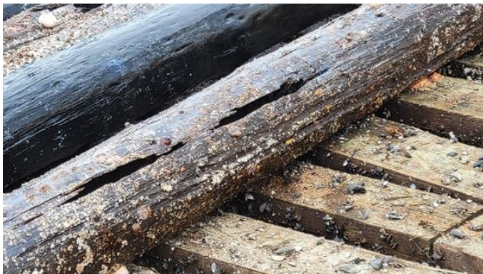
230. No 4 pile 4 th cluster – hollow core
