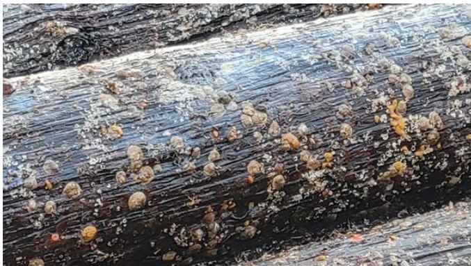
238. No 29 fender pile – generally satisfactory with light surface checking
