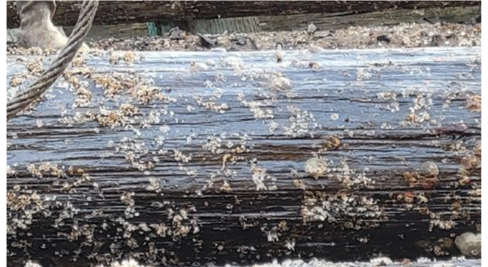
241. No 28 fender pile – generally satisfactory with light surface checking
