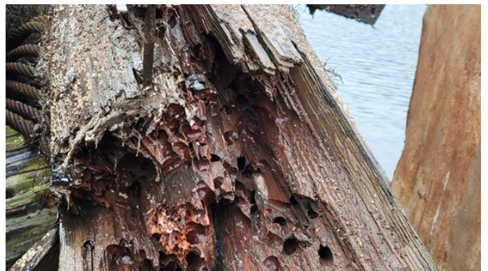
187. No 3 pile cluster – worm tracks
