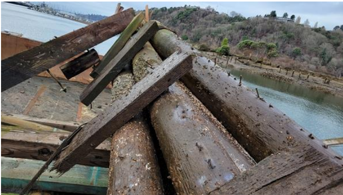
184. No 3 pile cluster
