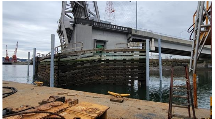
111. All temporary piles in position
