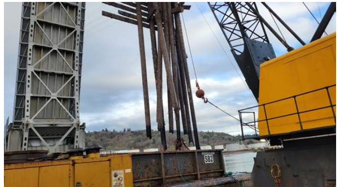
191. Lift and remove no. 2 pile cluster
