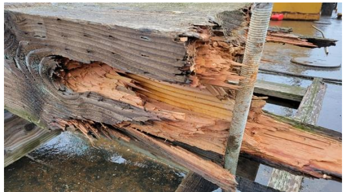
119. Catwalk condition of timber
