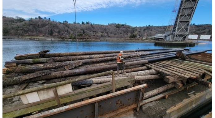
217. Pile Nos. 1-6 loaded on barge
