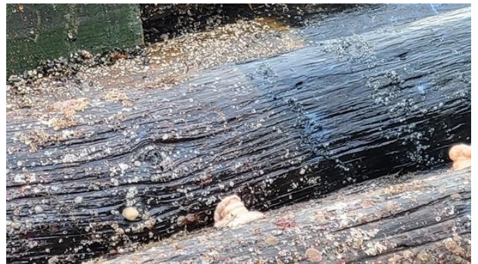
231. No 6 pile 4 th cluster – heavy worm tracks
