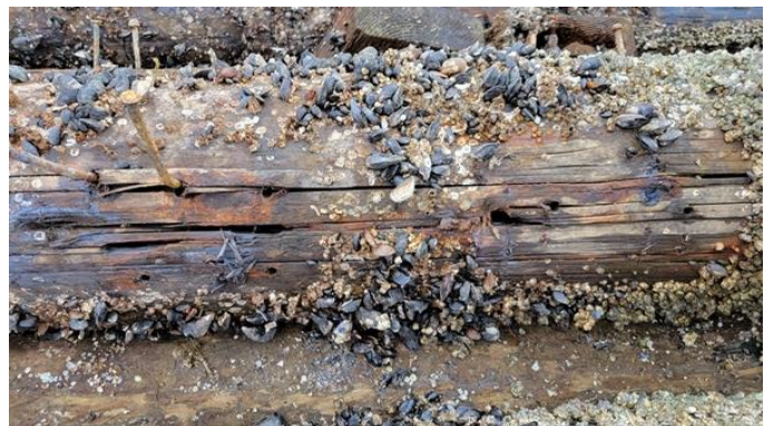
221. Surface checking and worm tracks
