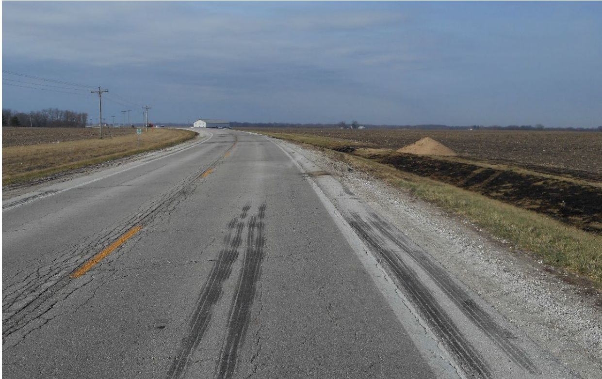
Figure 1. View looking west at tire marks leading to the area of impact.
