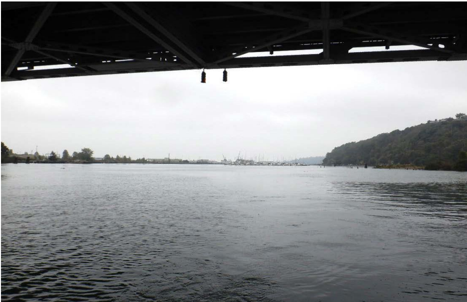
PHOTO No. 16 : Hylebos Bridge Edge, Looking Northwest.
