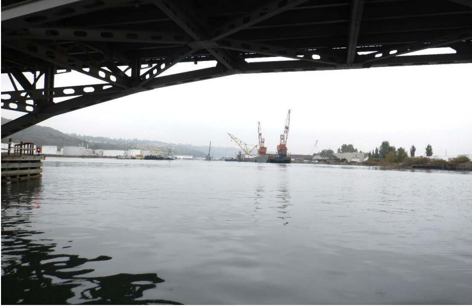
PHOTO No. 15: Hylebos Bridge Edge, Looking Southeast.
