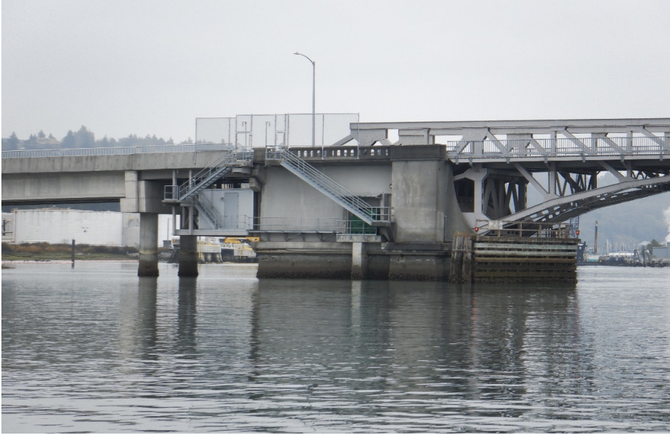
PHOTO No. 5 : Pier 5 and Pier 6, Looking Southeast - Note Pier 6 supported by two concrete columns and Pier 5, the Bascule pier, both located on the eastern side of the channel. Also note the protective timber fender system along the channel side of Pier 5.
