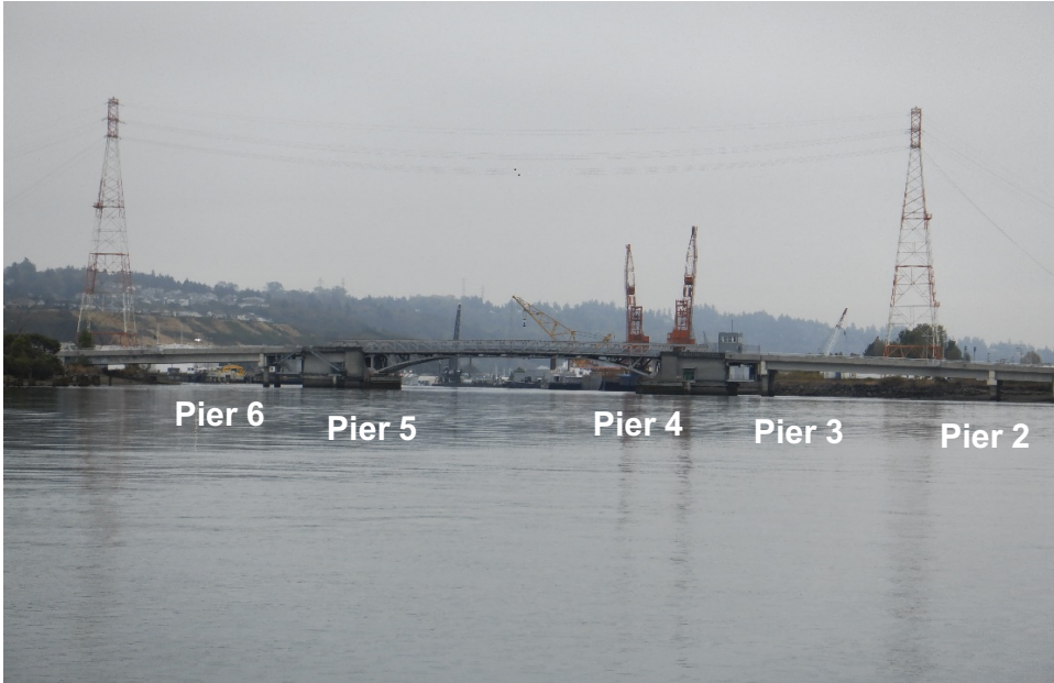
PHOTO No. 1 : Hylebos Bridge, Looking Southwest - The bridge is a double leaf trunnion bascule bridge with an approach located on the west and the east side of the span. Stationing for the structure and numbering of the substructure piers has been designated from west to east.
