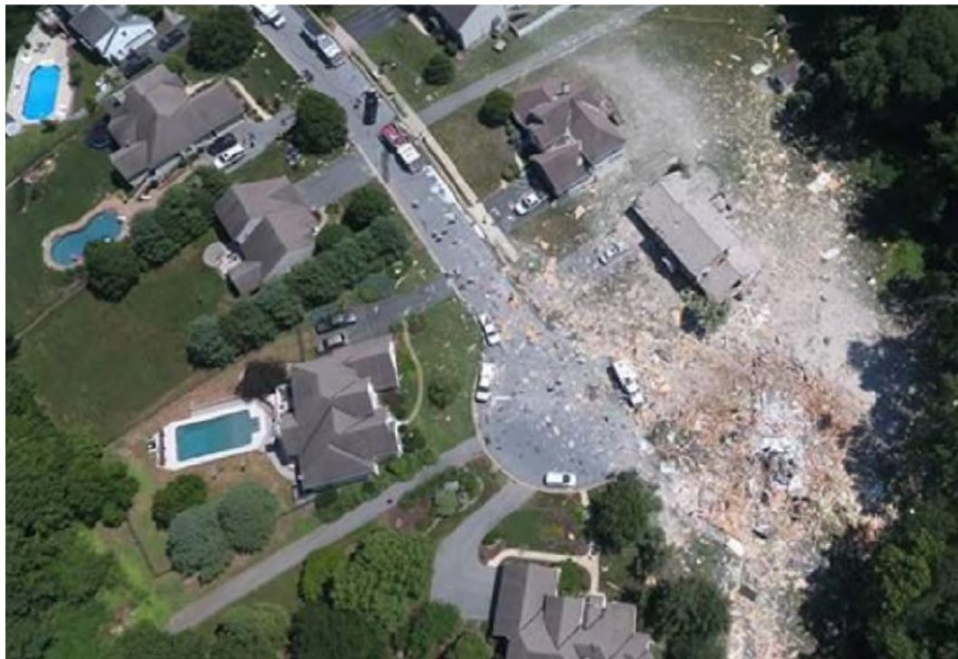
Figure 1. Debris field at cul-de-sac area where the explosion the occurred
