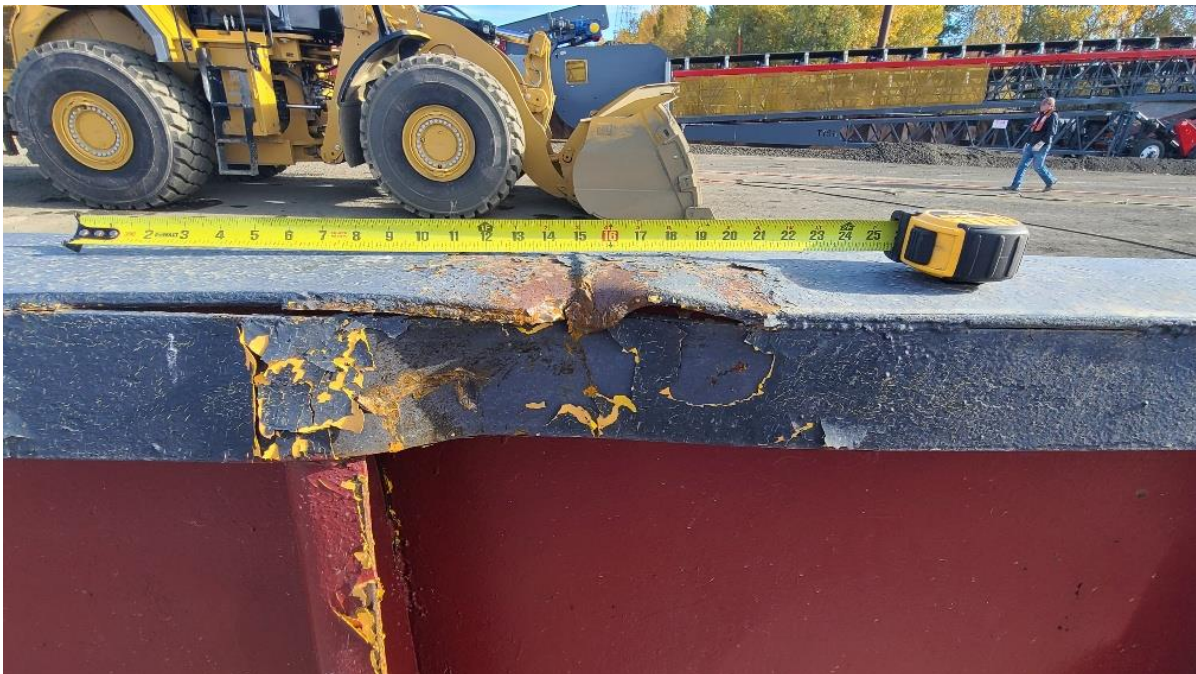
Damage to starboard coaming cap rail
