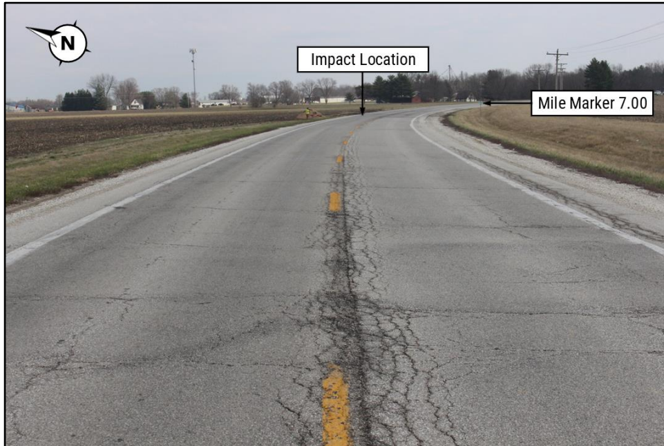
Figure 3. View from the centerline of US-24 facing in an easterly direction.
