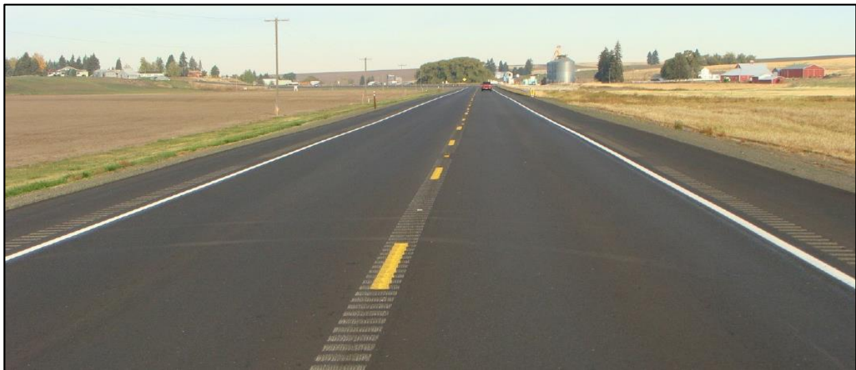
Figure 13. Example of milled CLRS and shoulder rumble strips. Source: FHWA
