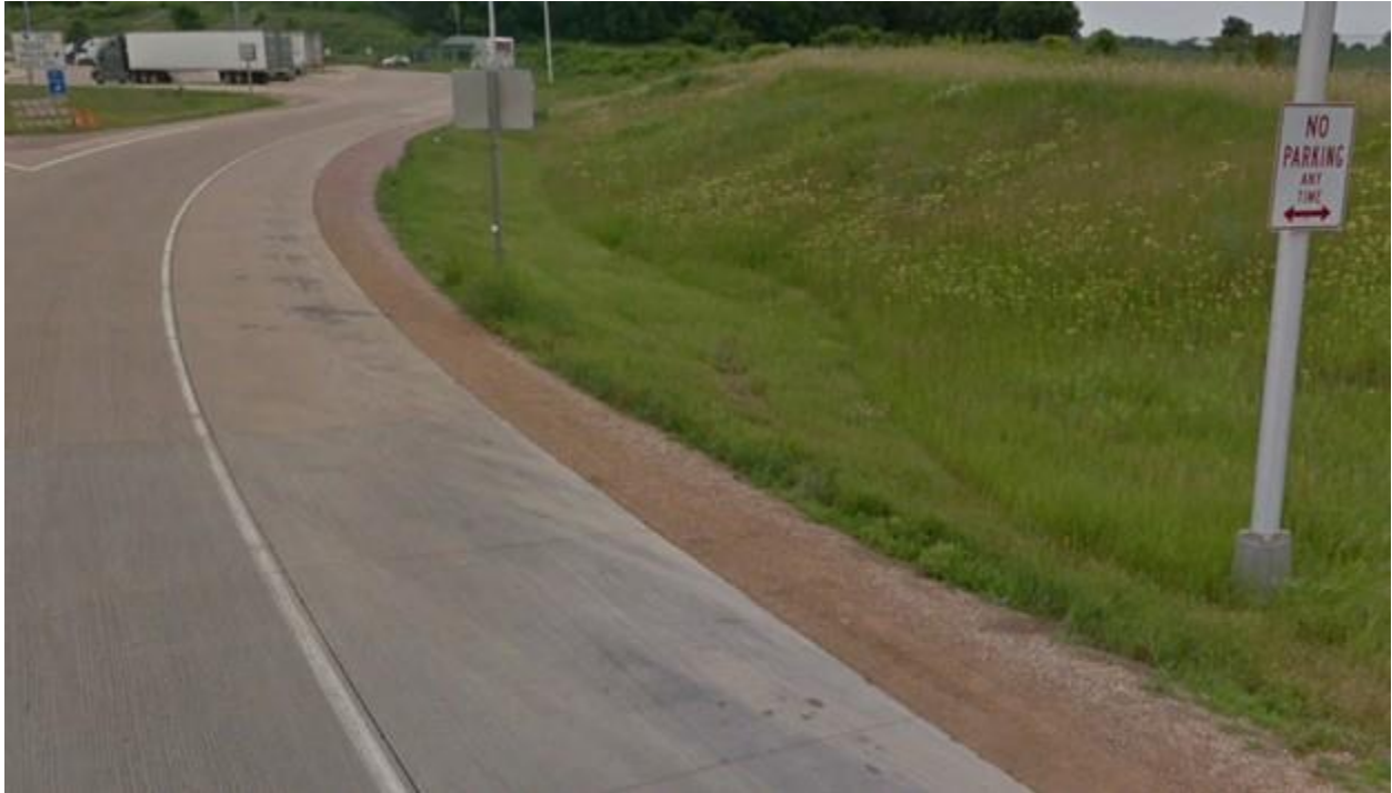
Highway Factors Photo 19 – View of the “No Parking Any Time” sign on the exit ramp to the Portage rest stop area northwest of Poynette, WI on I-90 (Source: Google Street Maps)
