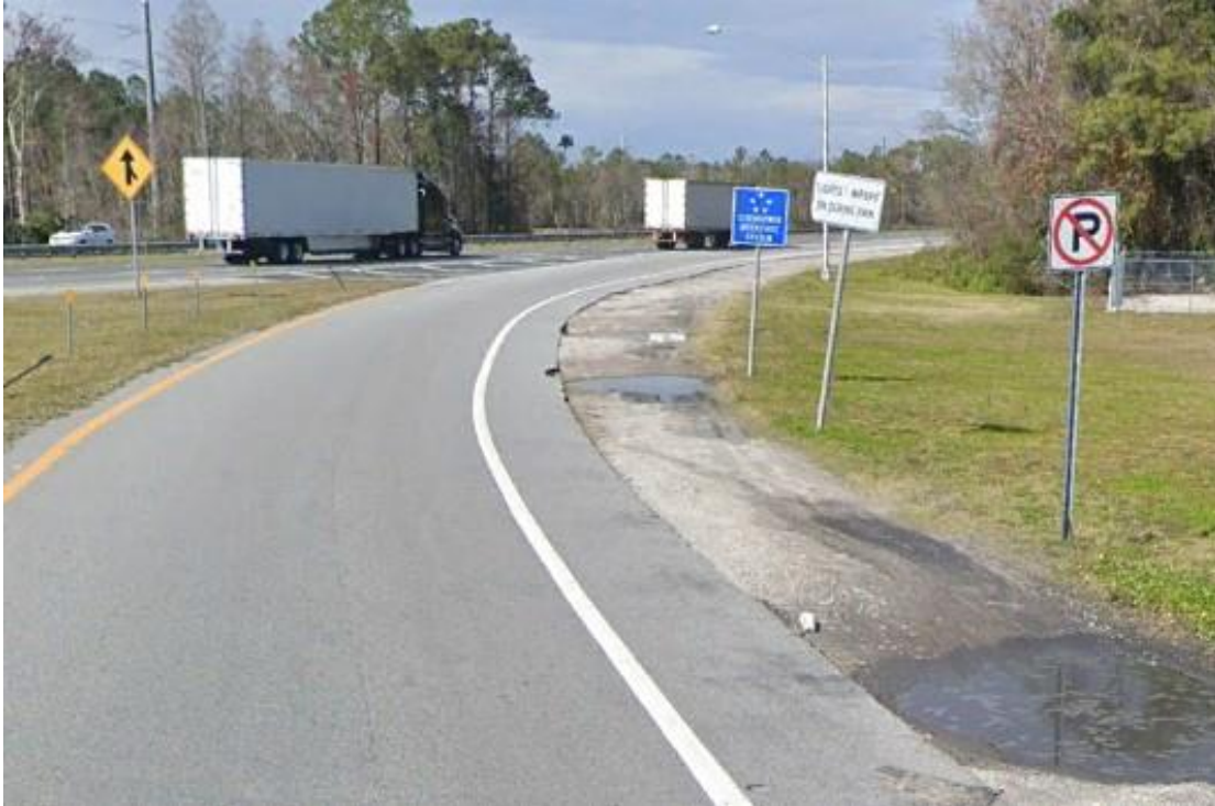
Highway Factors Photo 15 – View of the no parking symbol sign on the entrance ramp from the rest stop area south of St. Augustine, FL on I-95 (Source: Google Street Maps)
