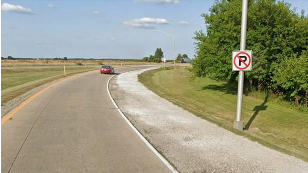
Highway Factors Photo 14 – View of the no parking symbol sign on the entrance ramp from the Spring Creek rest stop area near Covington, IN on I-74 (Source: Google Street Maps)
