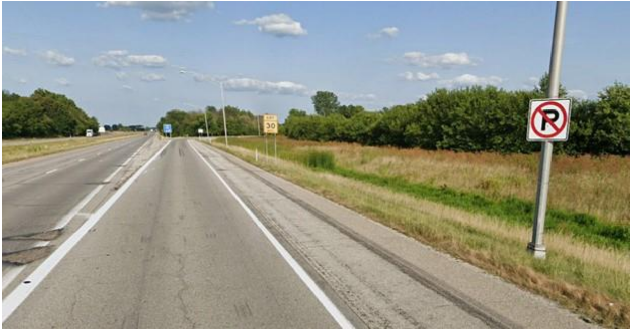
Highway Factors Photo 13 – View of the no parking symbol sign on the exit ramp to the Spring Creek rest stop area near Covington, IN on I-74 (Source: Google Street Maps)
