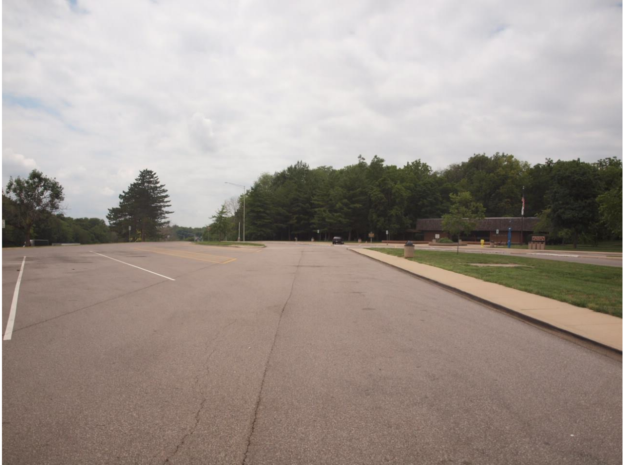
Highway Factors Photo 12 – View of the westbound Silver Lake rest stop parking lot standing in the aisle adjacent to the truck parking spaces looking to the west with the rest stop building located in the background
