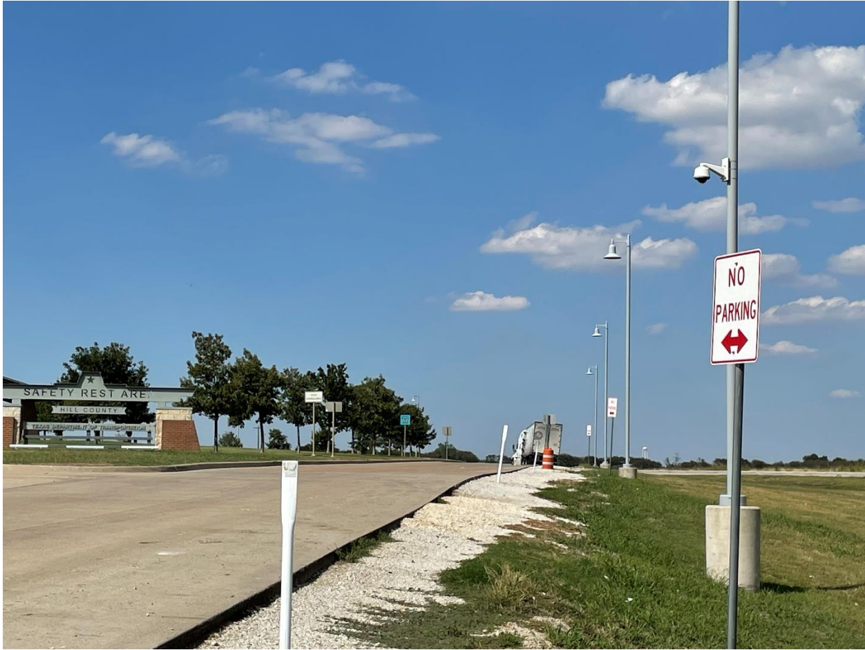
Highway Factors Photo 17 – View of the “No Parking” sign on the exit ramp and flexible delineator posts on the shoulder to the Hill County safety rest area south of Hillsboro, Texas on I-35
