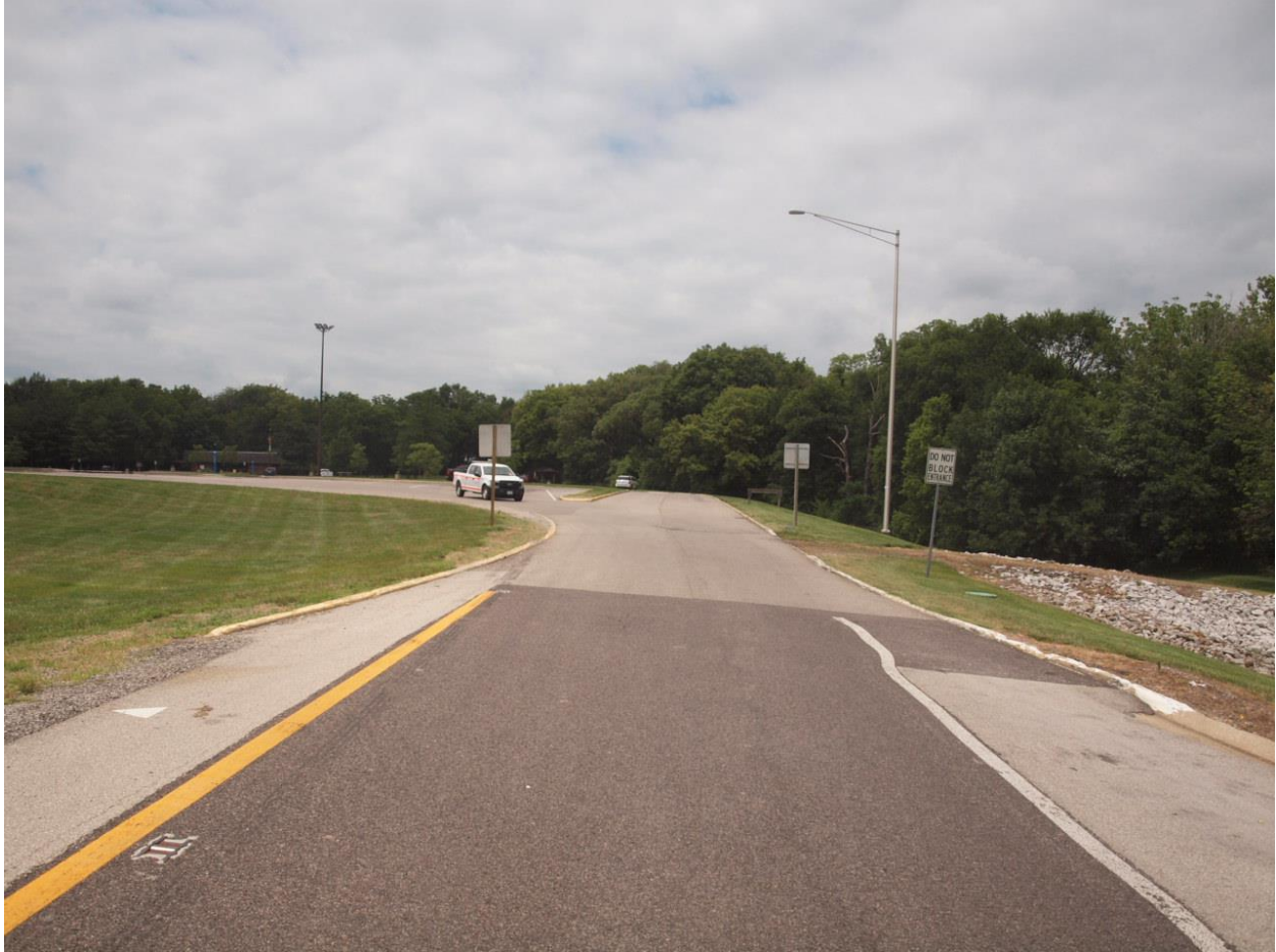
Highway Factors Photo 10 – View of the exit ramp to the westbound Silver Lake rest stop west of the crash location standing on the exit ramp looking to the northwest with the rest stop parking lot and building located in the background
