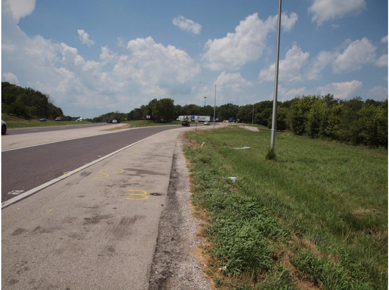
Highway Factors Photo 4 – View of the exit ramp to the westbound Silver Lake rest stop in the vicinity of the crash location standing on the edge of the paved right shoulder looking to the west
