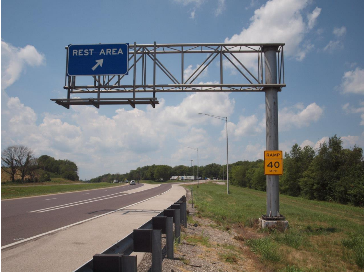
Highway Factors Photo 3 – View of the 40-mph advisory speed limit sign for the exit ramp to the westbound Silver Lake rest stop posted approximately 350 feet prior to the crash looking to the west
