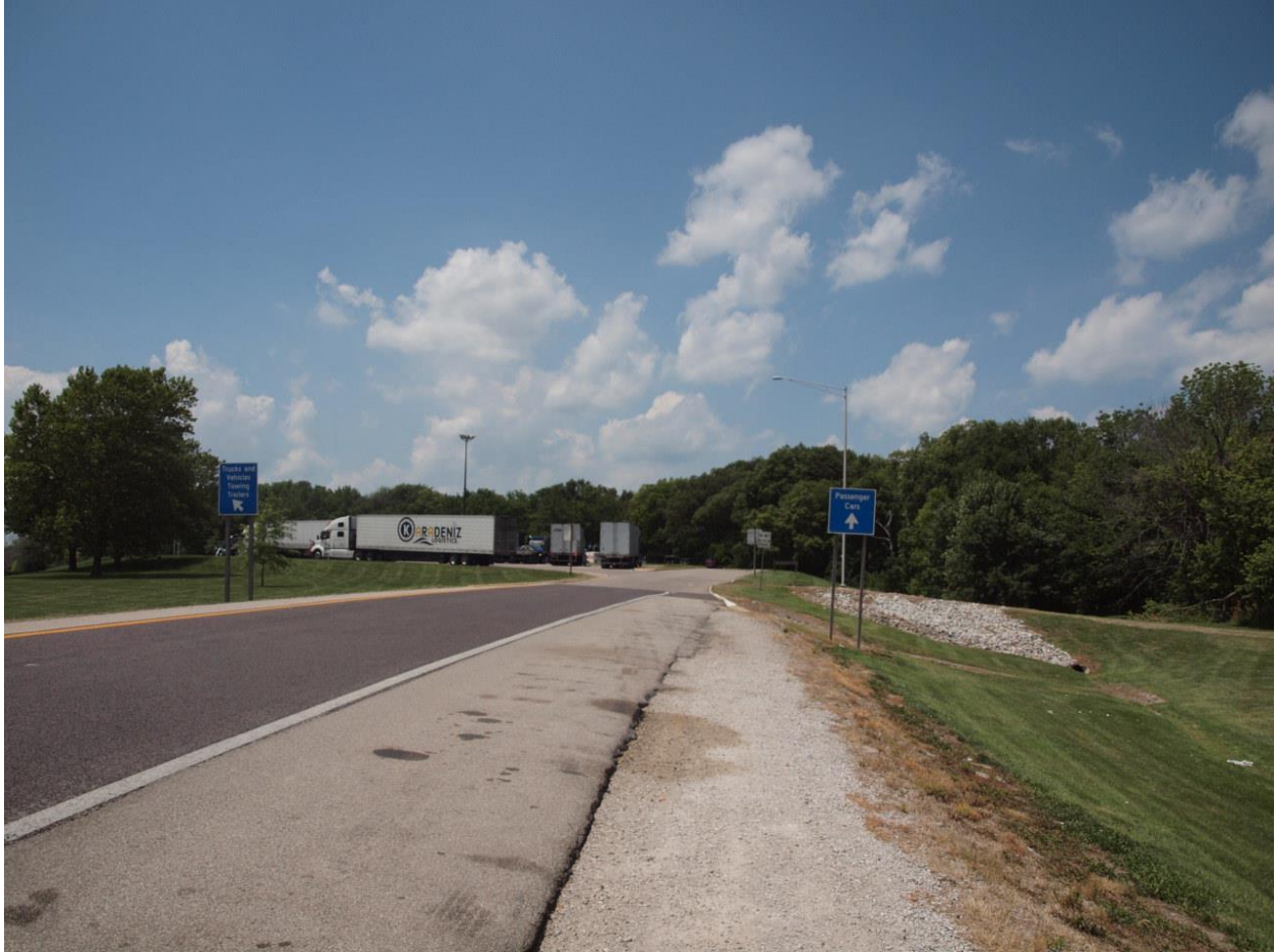
Highway Factors Photo 9 – View of the exit ramp to the westbound Silver Lake rest stop west of the crash location standing on the edge of the paved right shoulder looking to the northwest with directional signs for “Passenger Cars” and “Trucks and Vehicles Towing Trailers” located in the background
