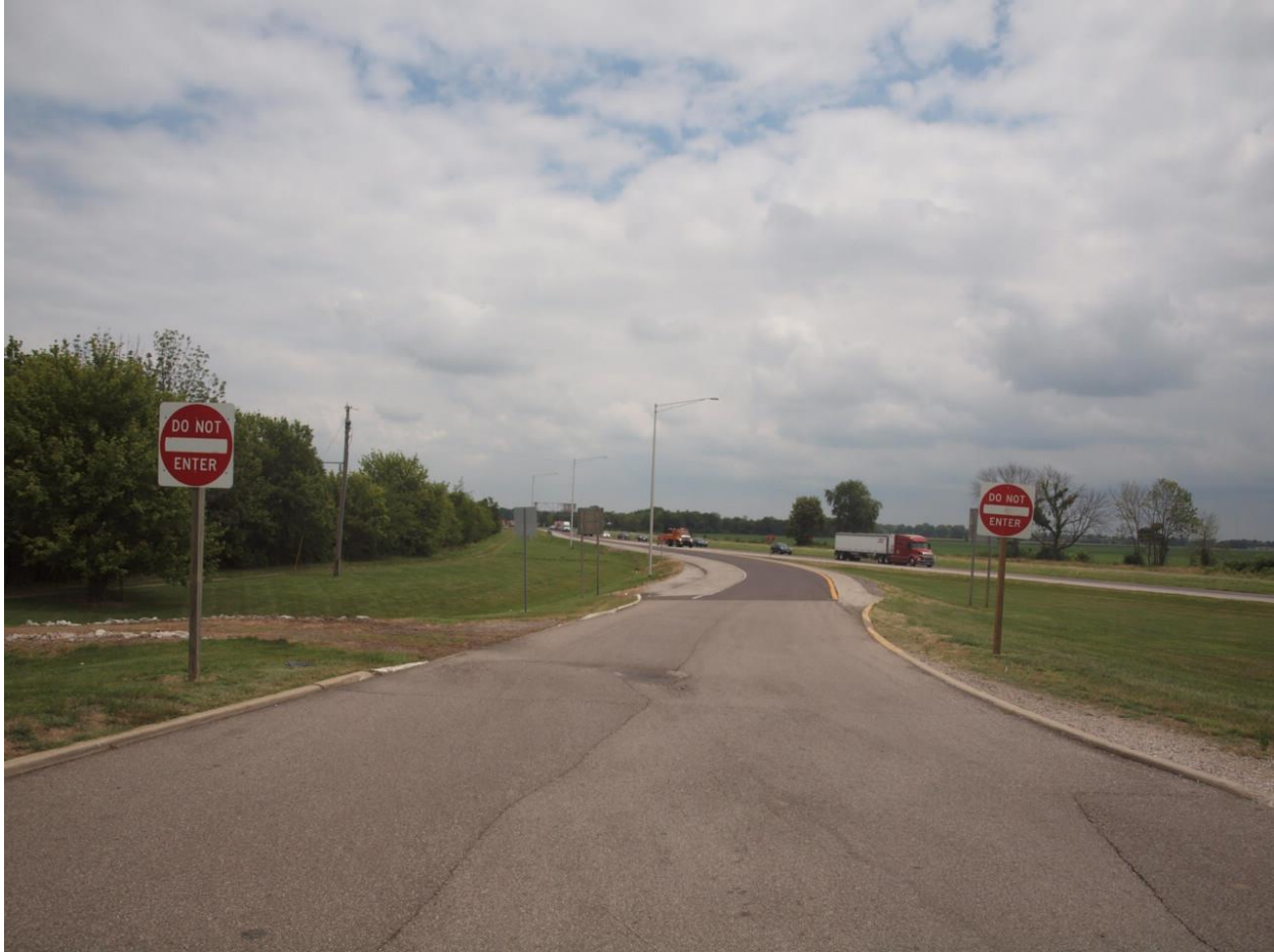
Highway Factors Photo 11 – View of the exit ramp to the westbound Silver Lake rest stop west of the crash location standing at the entrance to the rest stop parking lot looking to the east with “Do Not Enter” signs located in the foreground
