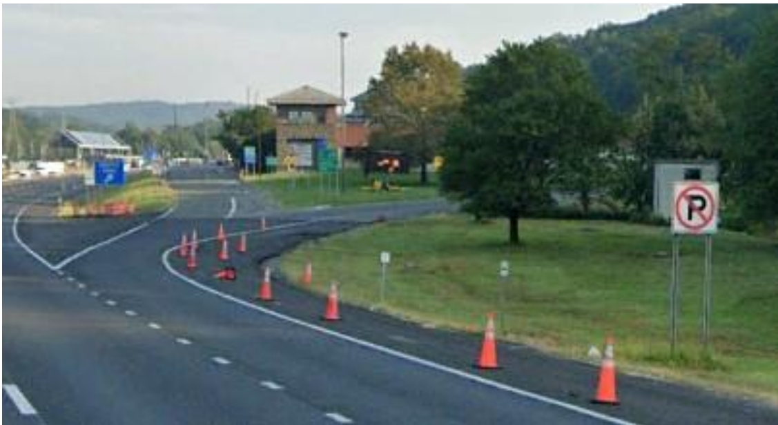
Highway Factors Photo 16 – View of the no parking symbol sign on the exit ramp and traffic cones on the shoulder to the Ramapo rest stop area near Sloatsburg, NY on I-87 (Source: Google Street Maps)
