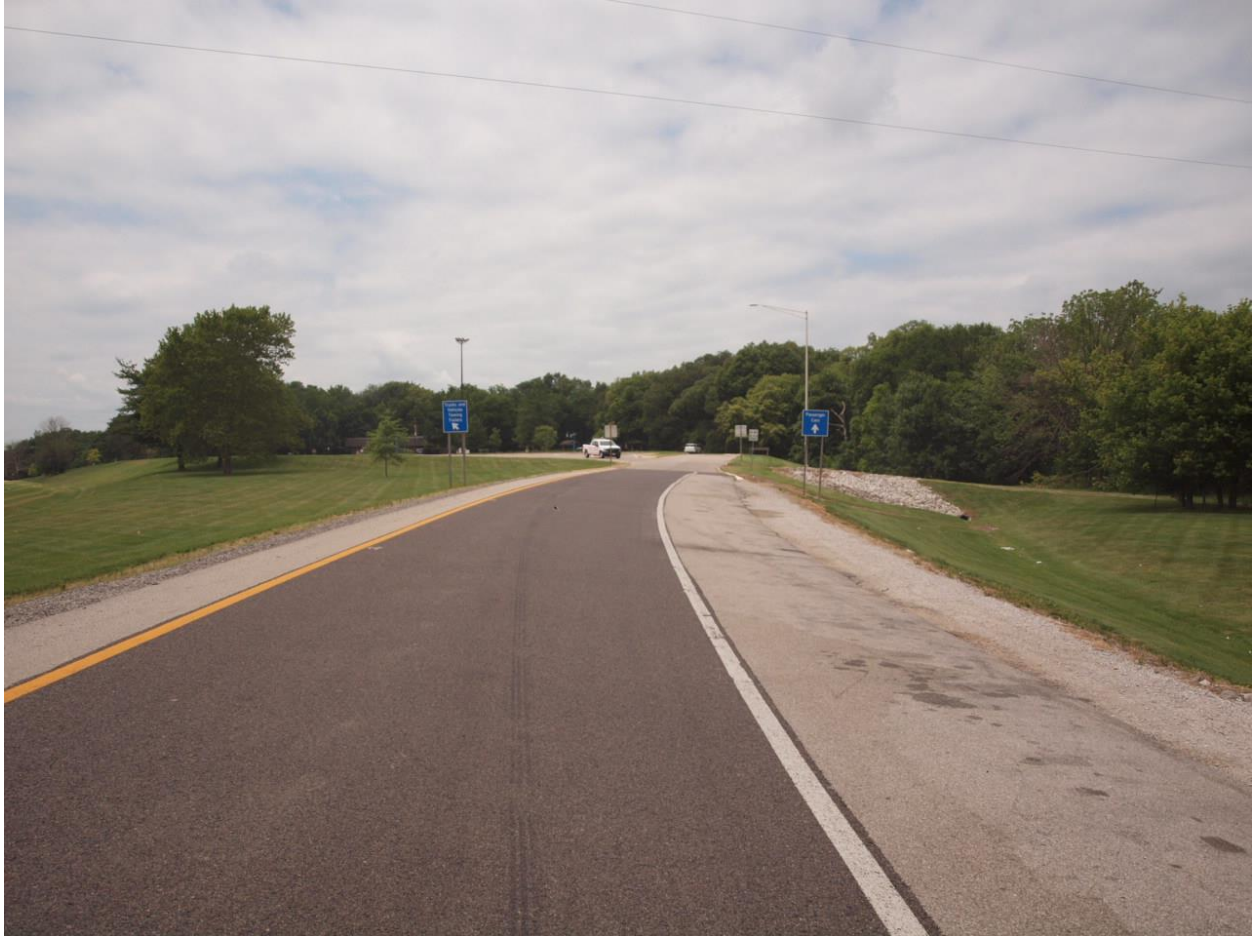
Highway Factors Photo 7 – View of the exit ramp to the westbound Silver Lake rest stop immediately west of the crash location standing on the exit ramp looking to the northwest
