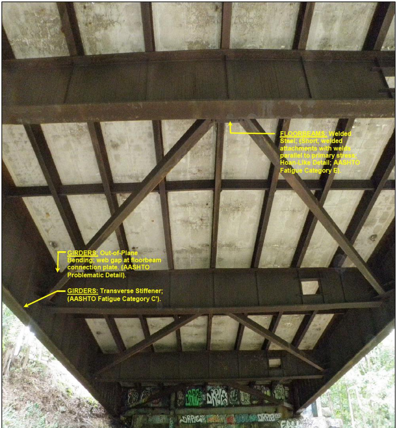
Photo 1 – Location of Fracture-Critical Members.
