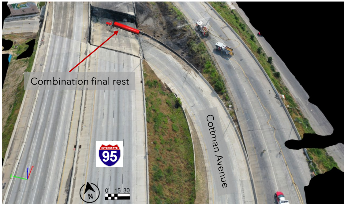
Figure 12. Image of the point cloud generated from the aerial photographs. Final rest of the overturned combination unit is noted. (Photos courtesy of PSP)
