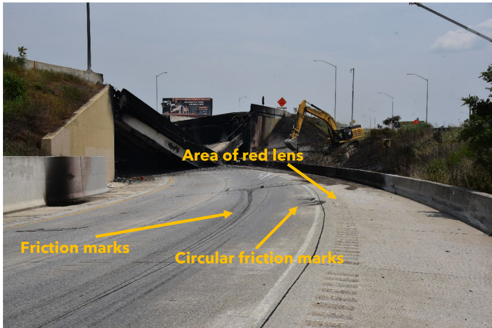
Figure 10. Photograph looking north along Cottman Avenue. In the photograph are the tire friction marks and noted is the area of the red lens and the beginning of the scorched concrete barrier. (Photo courtesy of PSP)
