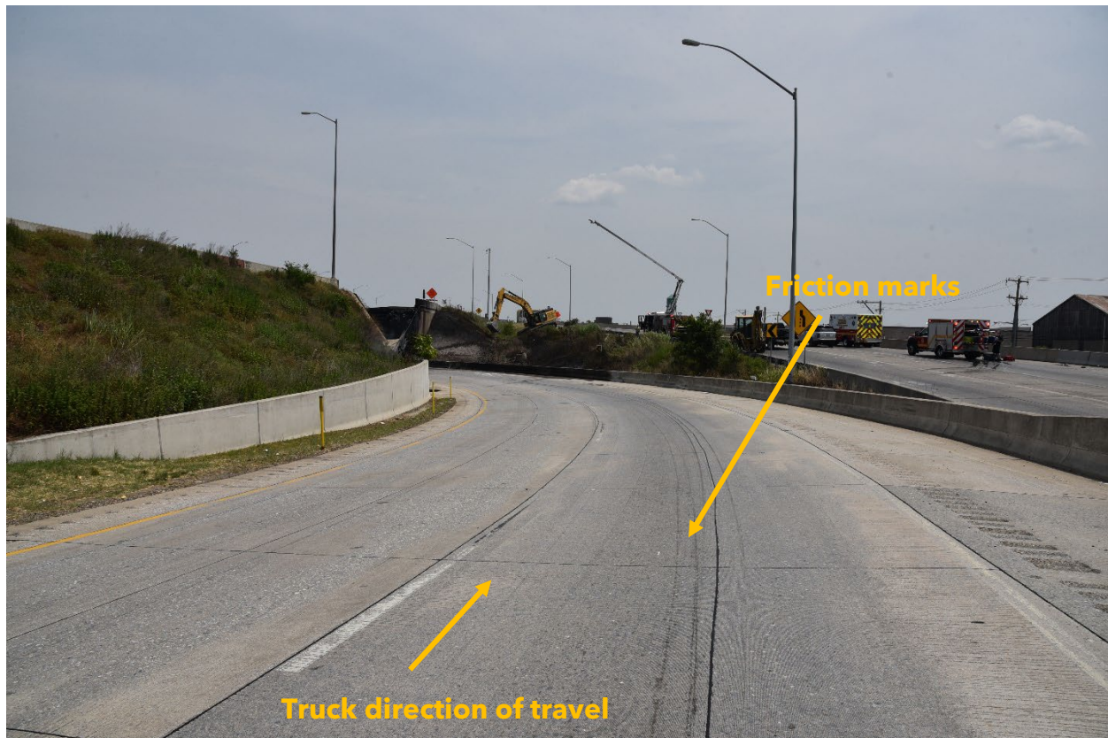
Figure 8. Photograph looking north along the Cottman Avenue off-ramp. In the photograph evidentiary marks are visible along the roadway, and concrete barrier. (Photograph courtesy of PSP)
