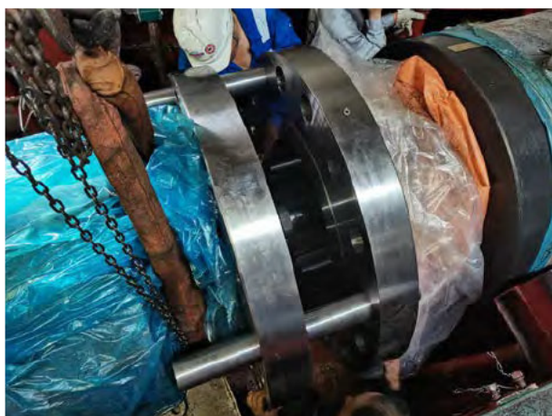
Make od shaft with coupling center
