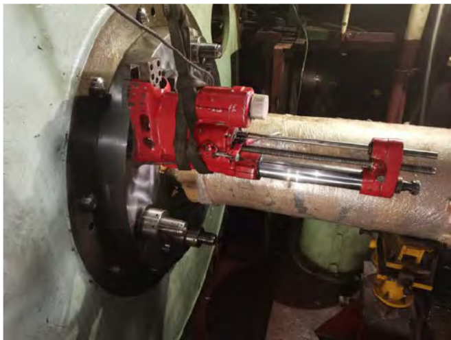
In-situ boring coupling holes
