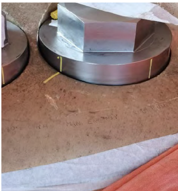
Check the rotation angle of bolt
