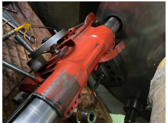
In-situ boring coupling holes
