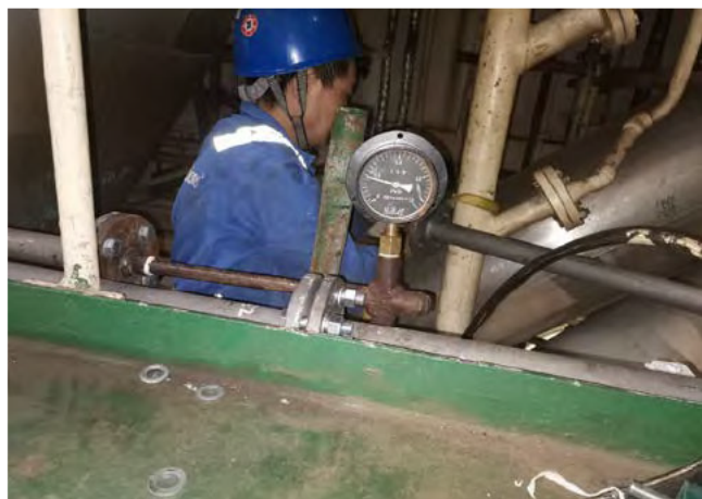
Presser test 3 bar
