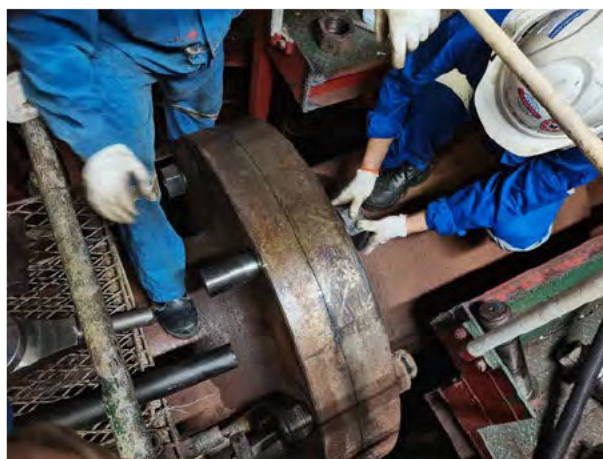
Removed AFT coupling bolts
