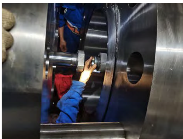
Installation internal connection pipe
