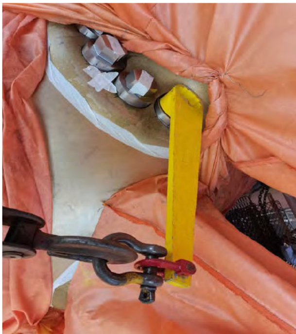
In accordance with instructions for tighten of bolt
