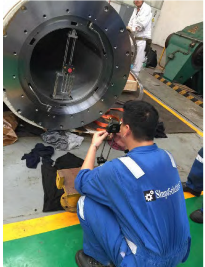
Alignment inspection with laser equipment
