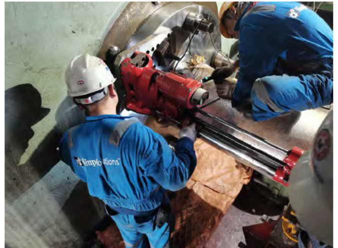
In-situ boring coupling holes
