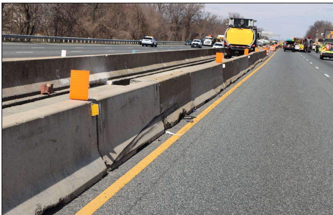
Figure 3: Photograph depicting evidence of Volkswagen contact with flexible concrete barrier (Maryland State Police - cropped).
