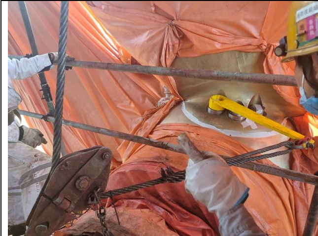
Cross tightened blade screws up to 500 Nm + 105 mm arc length 1 st time.
