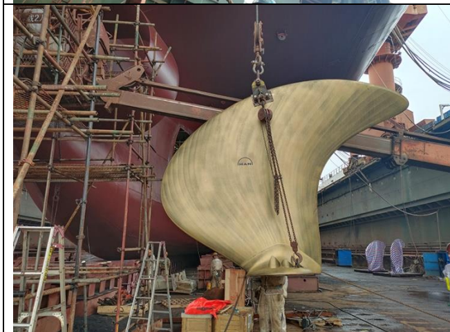
Lifted up propeller blade above to propeller hub.
