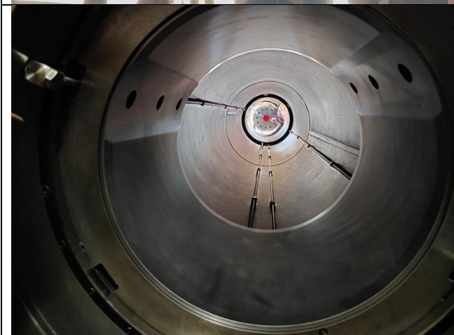
Well cleaned stern tub.
