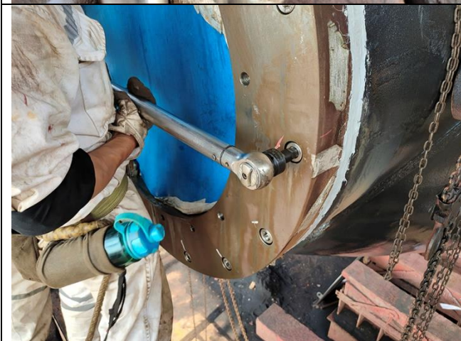
Cross tightened screws (Pos. 104) up to 340 Nm and lubrication with MOLYCOTE GN+.
