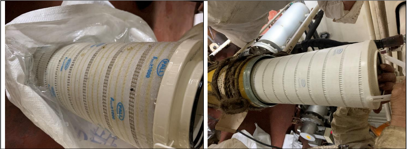
Flushing filters checked and replaced
