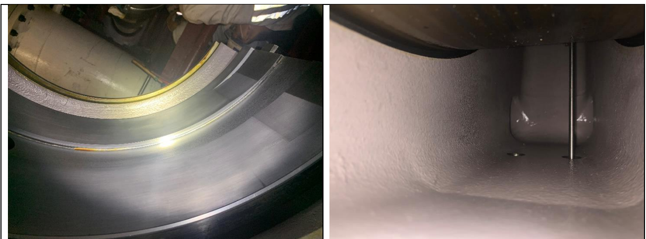
Intermediate shaft bearing cleaning condition checked
