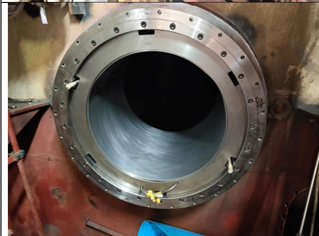
Installed adaptor flange.
