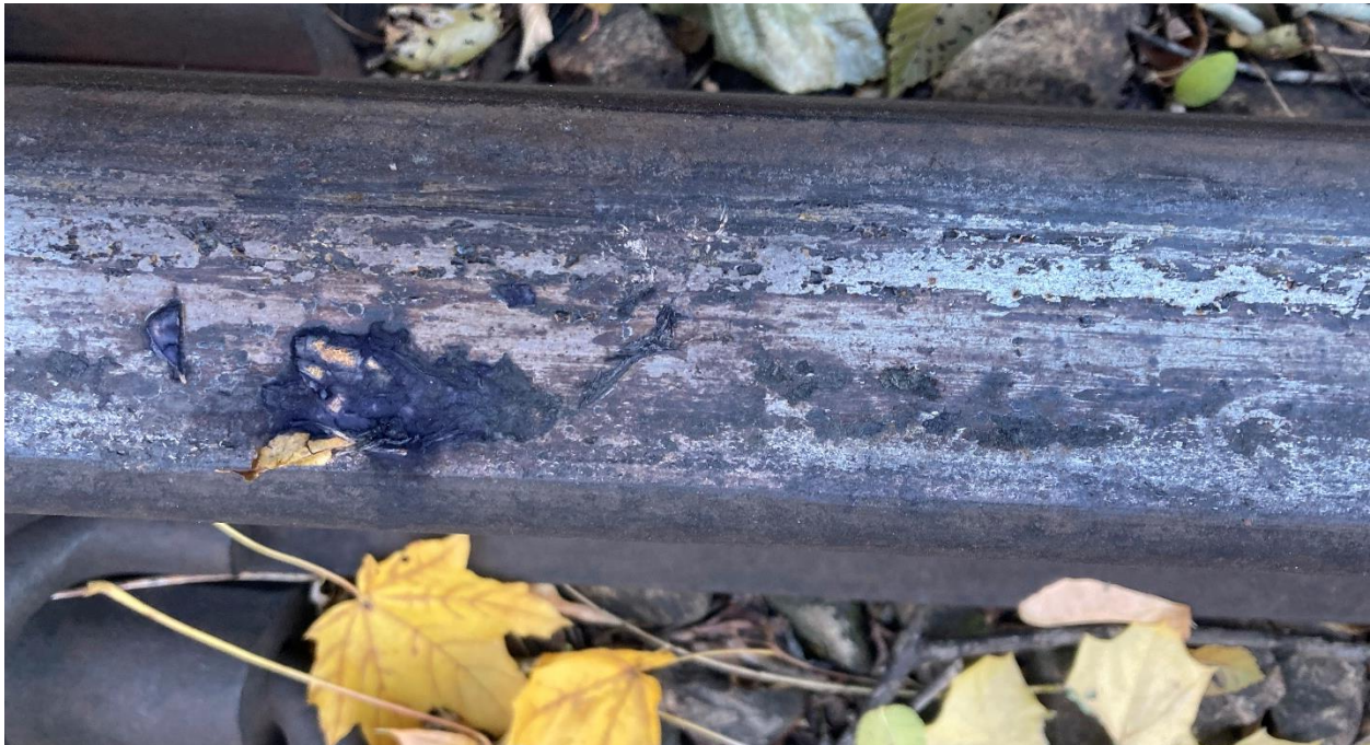
Figure #14: Leaf Residue on Top of Rail Approaching Accident Location
