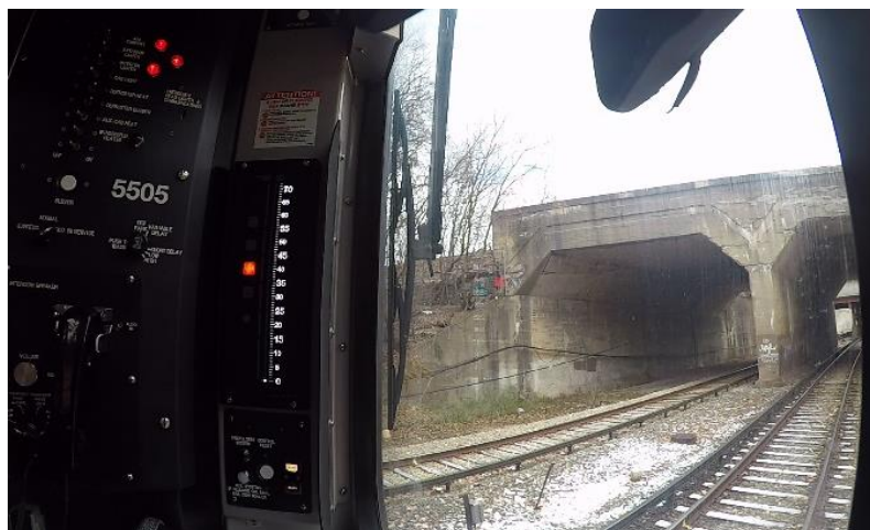
Figure #4: Test Run #1 – Location where train came to a stop
