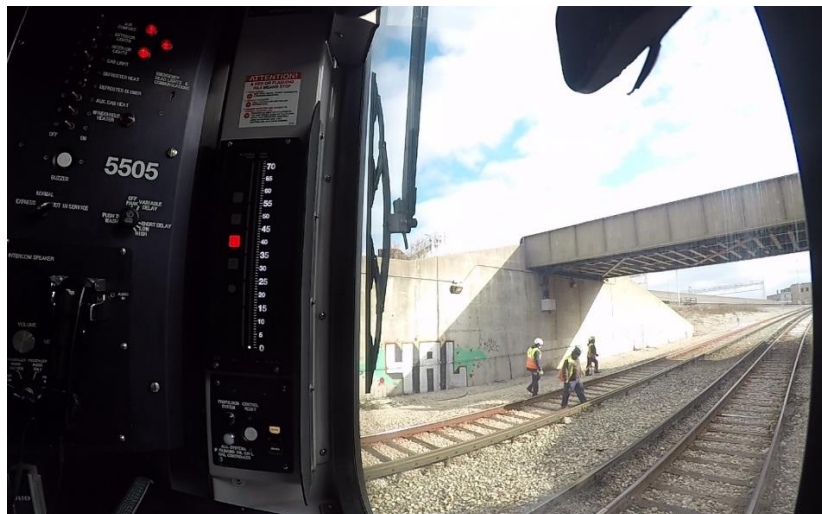
Figure #8: Test Run #2-Take 2 – Location where train came to a stop
