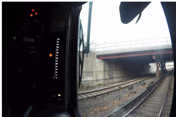
Figure #28: Test Run #10 – Location where train came to a stop
