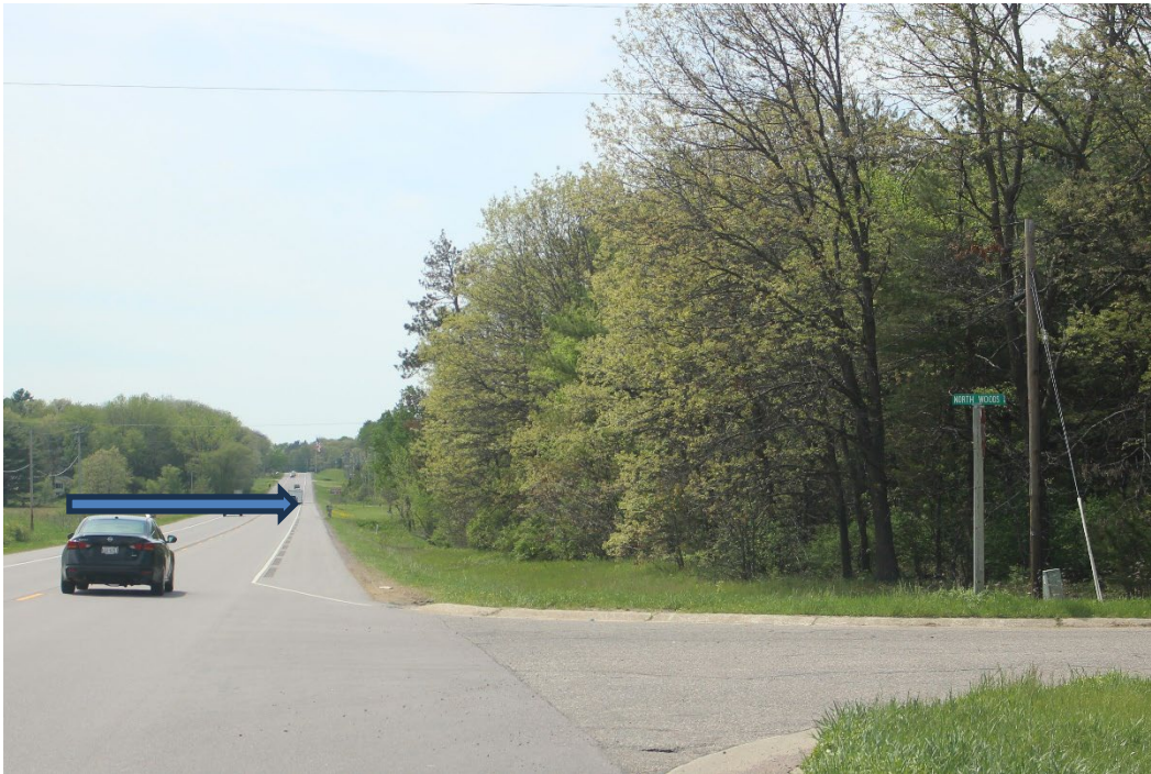
PHOTO 1: Looking Westbound on Wisconsin State Route 33.( Source: NTSB)
