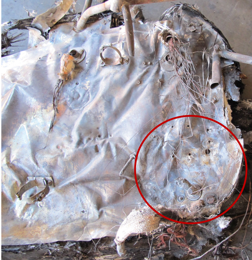
Figure 3. The right side of the fire wall. Thermal damage highlighted by red circle.
