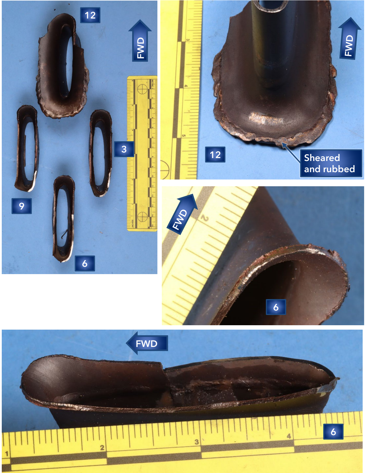
Figure 26. Inner ends of the inner struts after cutting from the bearing housing support (upper left). Closer views of fractures through the inner strut inner flanges at the 12 o'clock (upper right) and 6 o'clock (lower right and lower center) positions.
