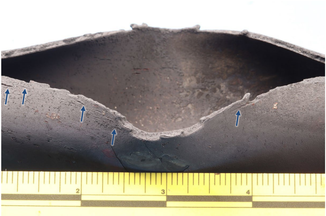
Figure 7. Oblique view of the pipe B fracture showing step features in the fracture plane corresponding to longitudinal crack-like pits (indicated with unlabeled arrows) on the exterior surface.
