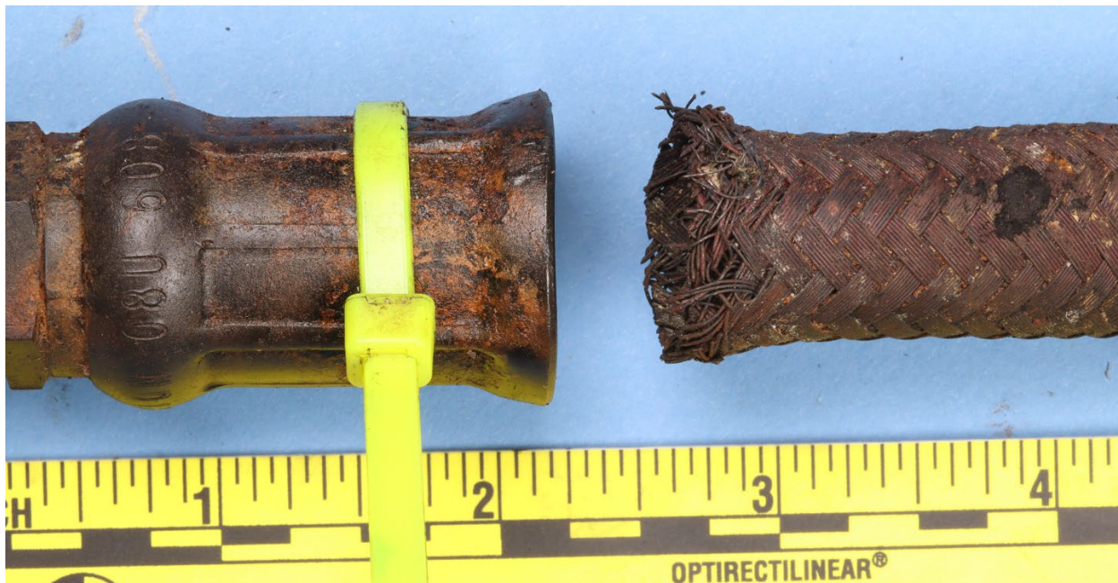
Figure 13. Close view of the separated end of the hose and corresponding crimped sleeve. The reinforcement braid adjacent to the cut end was disturbed and splayed slightly outward within 3/8 inch of the end face.
