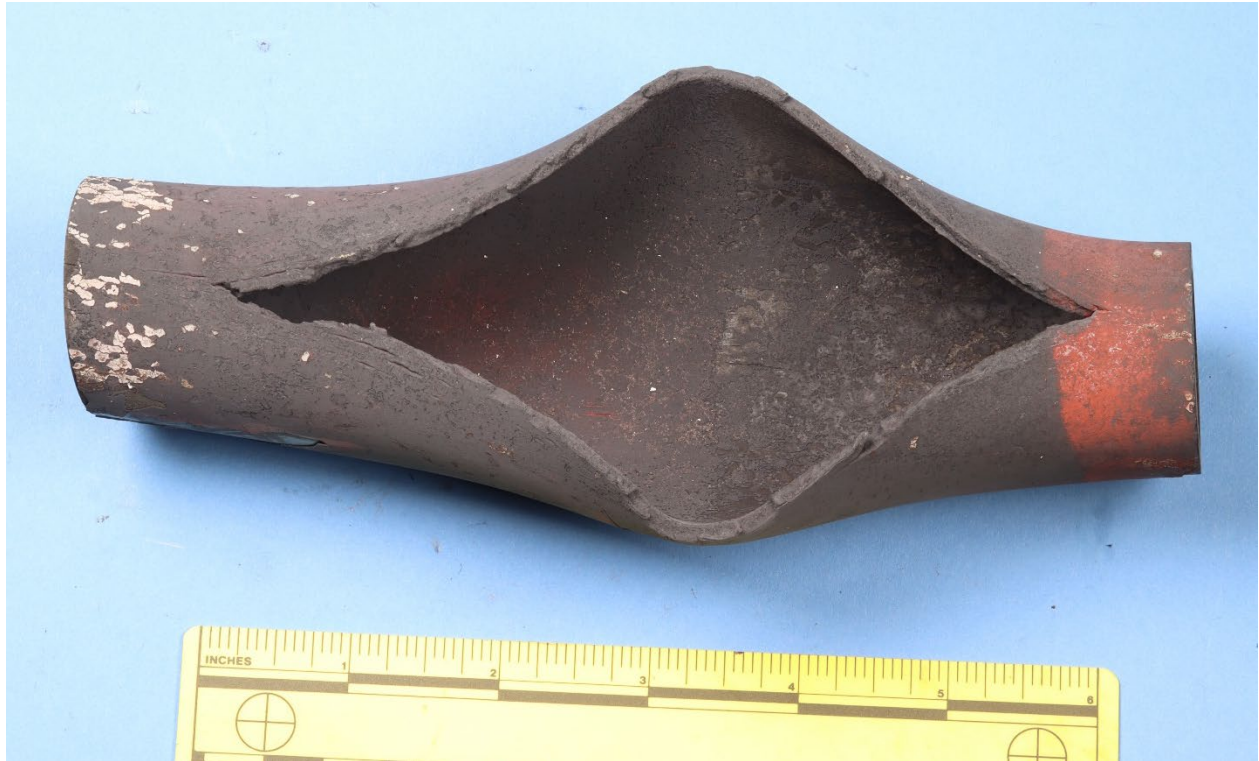
Figure 6. Close view of the pipe B fracture after sectioning and partial deoxidation.
