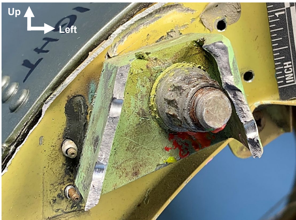
Figure 12. View of the fractured upper right fitting.
