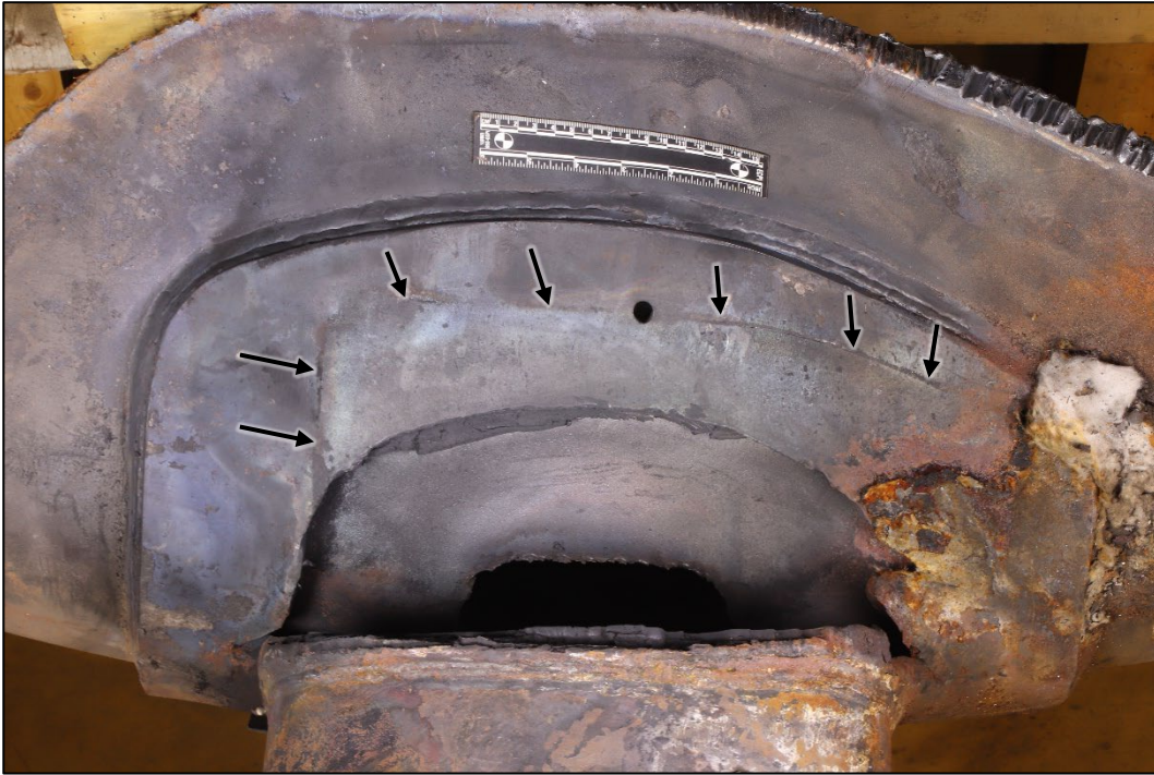
Figure 4. Contact mark on the front sill pad (unlabeled arrows) corresponding to contact with the jacket opening for the stub sill.
