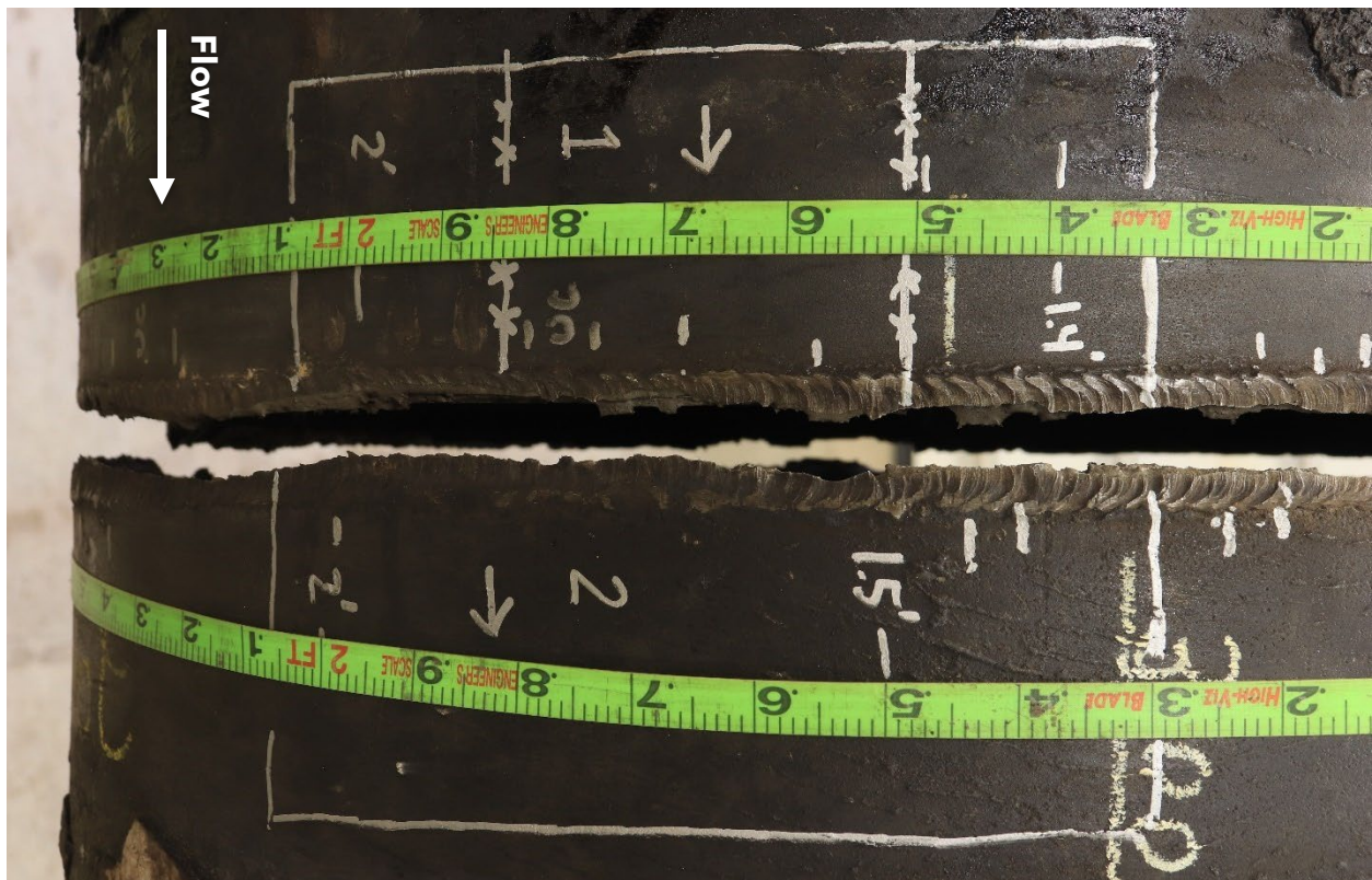
Figure 8. Mating fracture surfaces along the girth weld between Pipes 1 and 2, showing areas to be sectioned.
