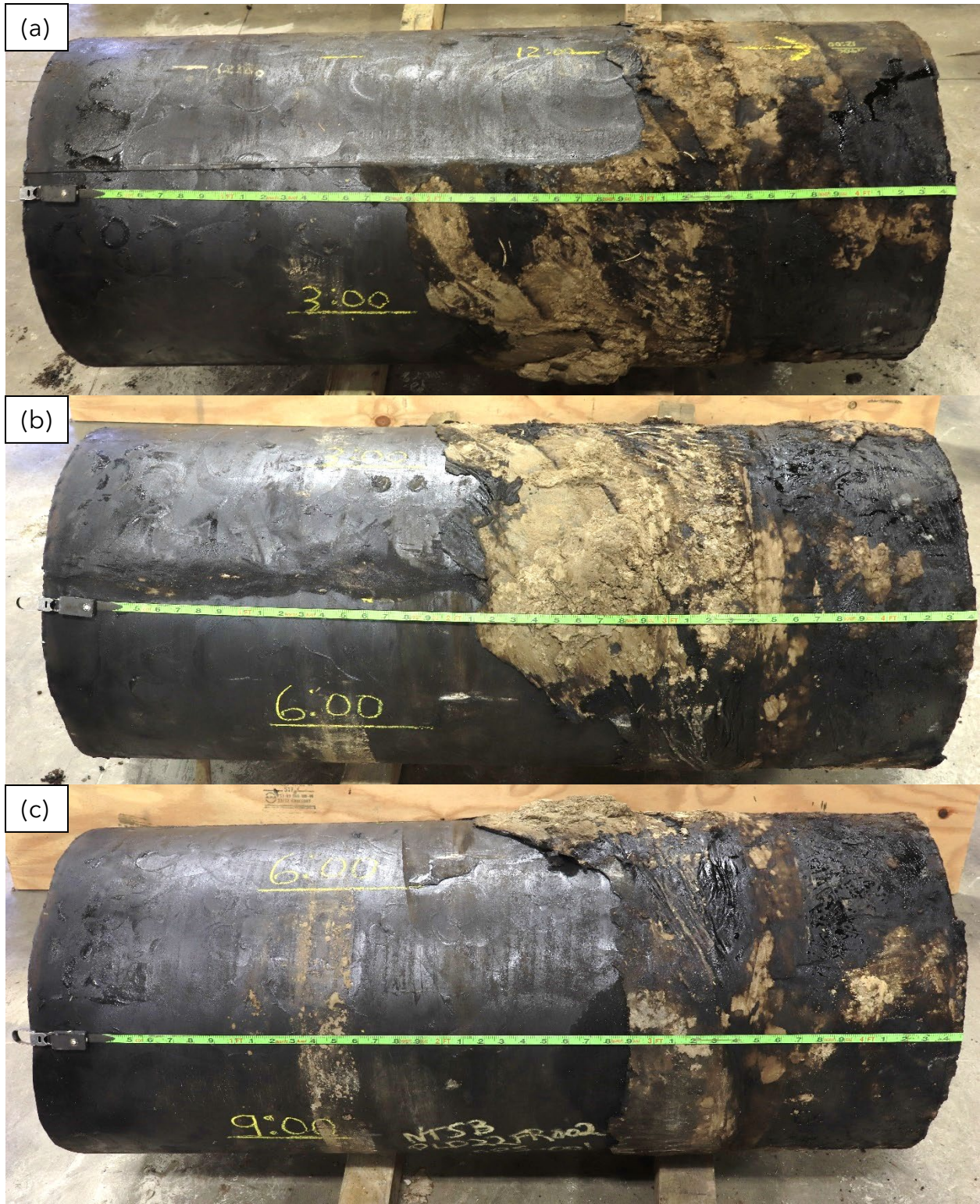
Figure 1. Views of the Pipe 1 pipeline section from three different views, as received at DNV.
