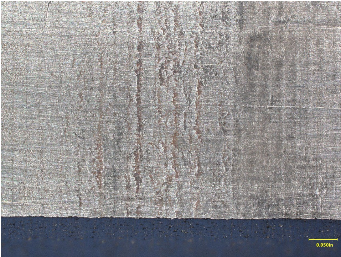
Figure 6. View of the most severe band of fretting wear on the axle wheel seat surface.
