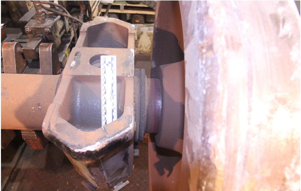
Figure 2. The gap between the inboard wheel face of the RS wheel and the axle seat hub.
